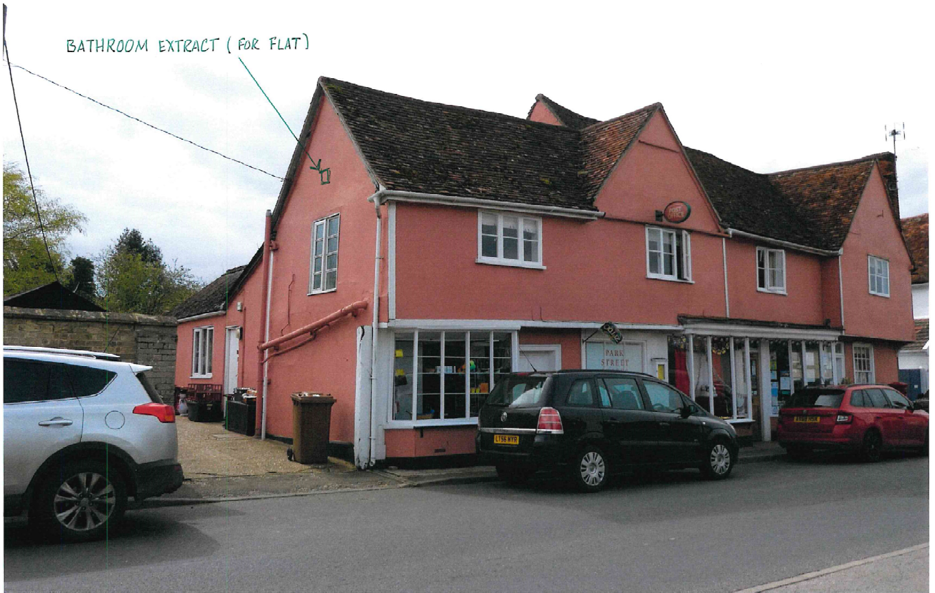
Bathroom (to flat) extract lead covered vent as seen from the side elevation
