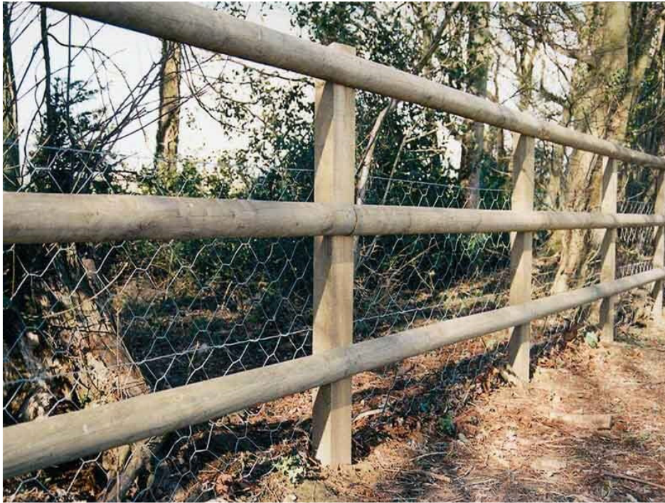
A typical example of the proposed post and rail timber fence approximately 1.2m high between the gardens and the driveway
