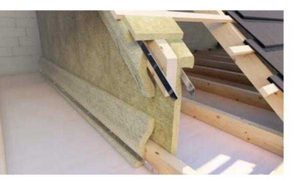
Preventing the spread of fire and inhibiting the passage of smoke in concealed spaces
