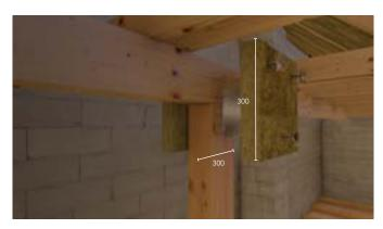
25mm thick ROCKWOOL BeamClad® fixed with FirePro Glue and nailed, or 50mm Fire Barrier secured with screws and large square washers. Use 50mm nails for BeamClad and 70mm screws for Fire Barrier.
