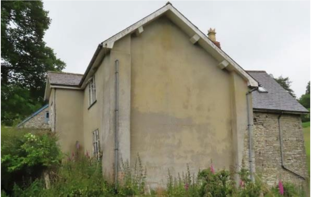
Photograph 3. House at Troedrhifedwen. Exterior. East elevation.
