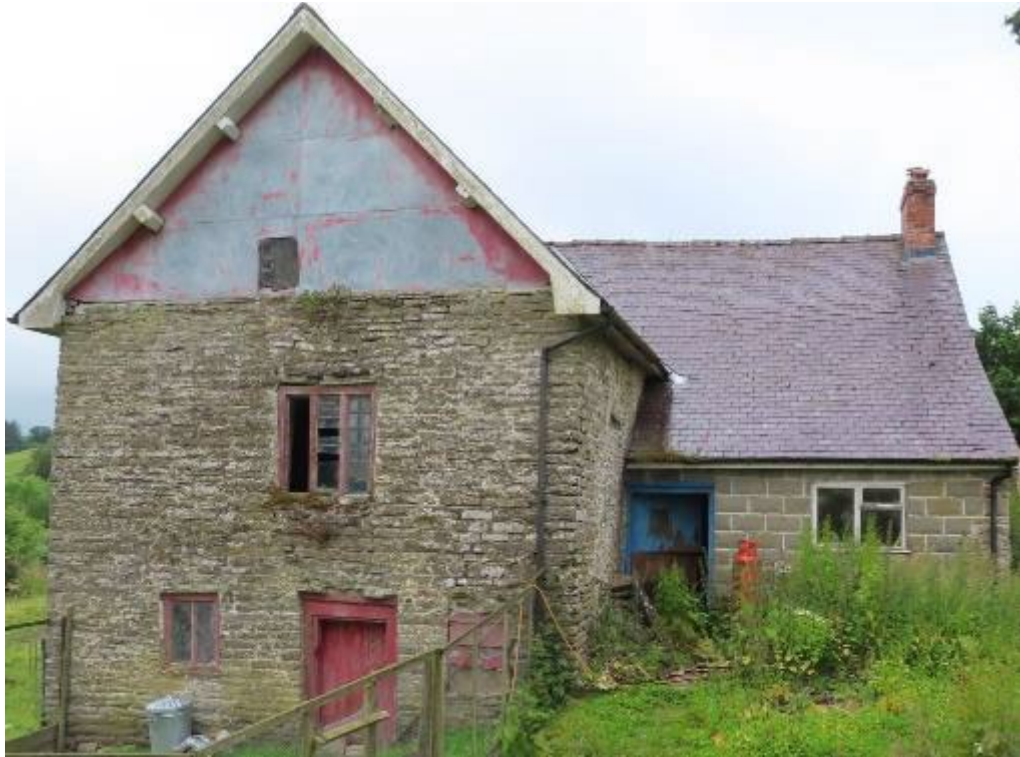
Photograph 1. House at Troedrhifedwen. Exterior. North elevation.
