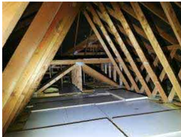
Photo 4. Showing the roof void over the main part of the building
