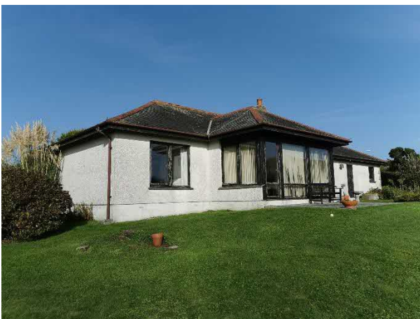
Photo 1. Showing the house from the south west
