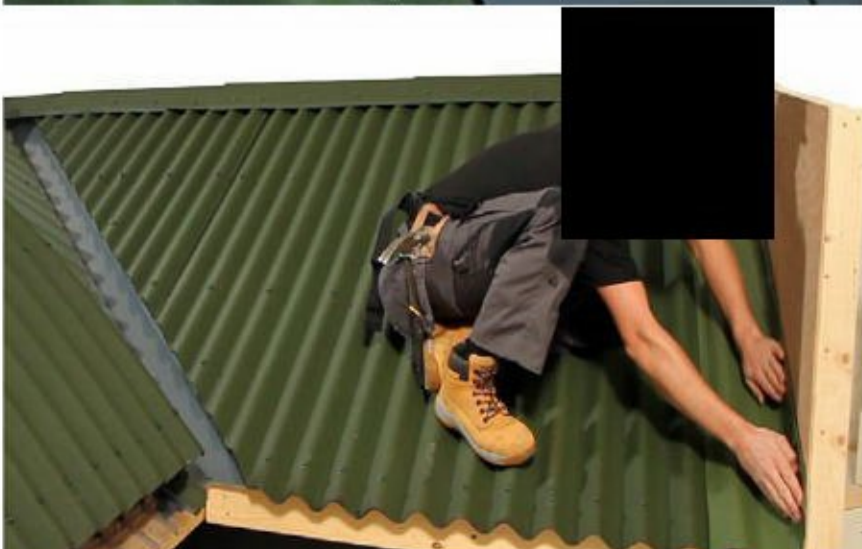
Side wall abutment Metal or preformed proprietary side wall abutments; or Onduband self-adhesive flashing tape are used to seal side wall abutments providing a minimum of 7.5 cm upturn against the wall and dressed over at least one full Onduline corrugation. Complete with a separate wall cover flashing.
