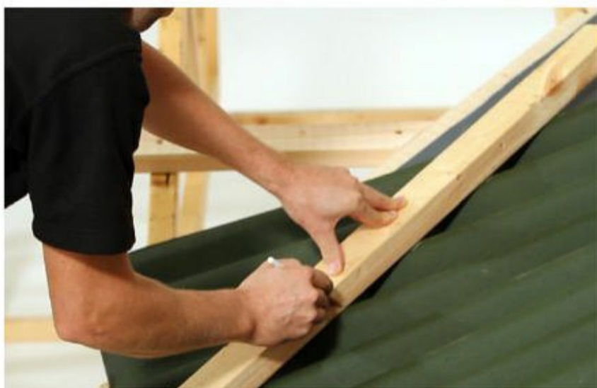
Marking sheet to valley Position the Onduline sheets up the line of the valley and mark out the cut line, allowing for a minimum of 4cm sheet drip edge into the valley gutter.
