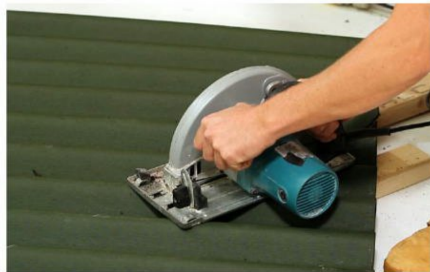
Cutting sheet Remove the sheets from the roof supporting either side of the required cut line, then use a mechanical saw to cut the sheets as required.
