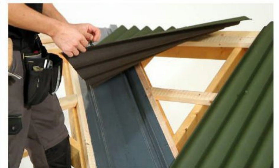
Positioning sheet The sheets are then positioned back on the roof, aligned square to the line of the roof sheets providing the minimum of 4cm drip edge into gutter.
