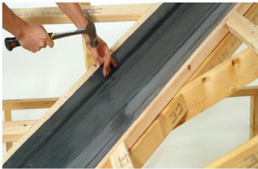
Fixing GRP valley lining Alternatively pre-formed GRP valley liners are laid between the purlin trimming battens and secured by nailing. Underlay can be dressed over the upstands.
