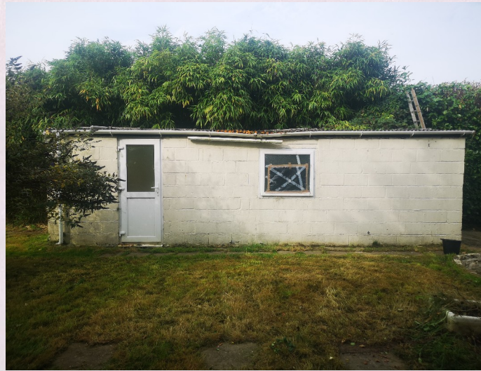
Photo of Existing Side Elevation (NTS)
