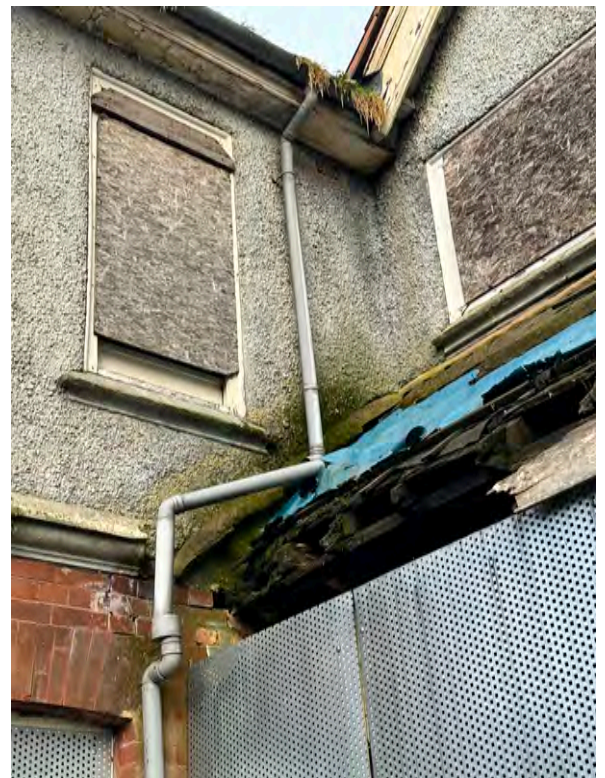
2.1.1.4 The small mono pitch roofs are also in poor condition, tiles have been removed and sheet material used to weather the pitch, this is not a robust permanent solution and, as is to be expected has failed.
