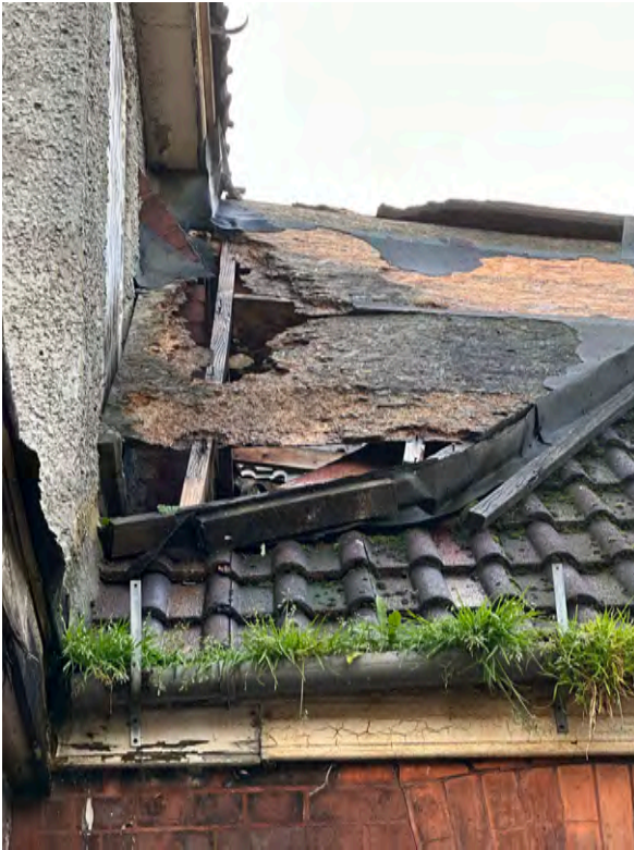
2.1.1.4 The small mono pitch roofs are also in poor condition, tiles have been removed and sheet material used to weather the pitch, this is not a robust permanent solution and, as is to be expected has failed.
