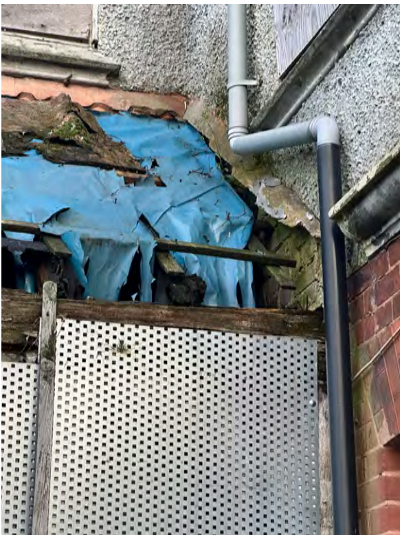
2.1.1.5 The flat roofs are felt covered, all are in poor condition.
