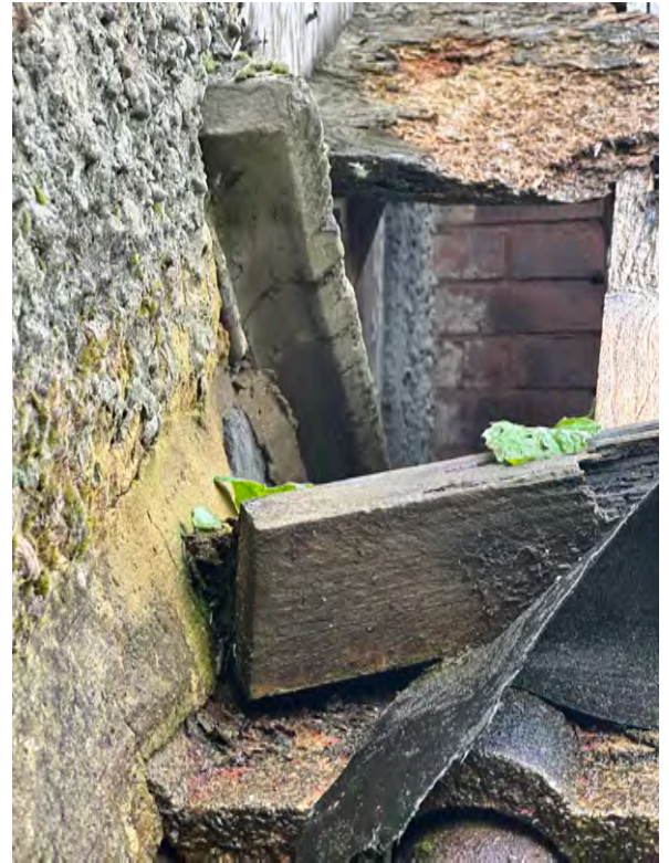
2.1.1.4 The small mono pitch roofs are also in poor condition, tiles have been removed and sheet material used to weather the pitch, this is not a robust permanent solution and, as is to be expected has failed.
