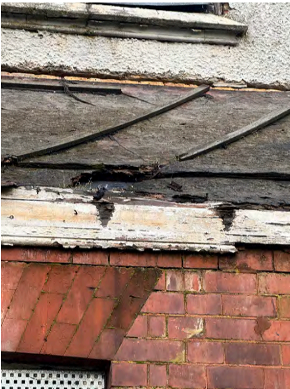
2.1.4.1 The gutters and down pipes are in poor condition, sections have failed and as such the discharge of rainwater is not being controlled and is therefore saturating the building fabric.
