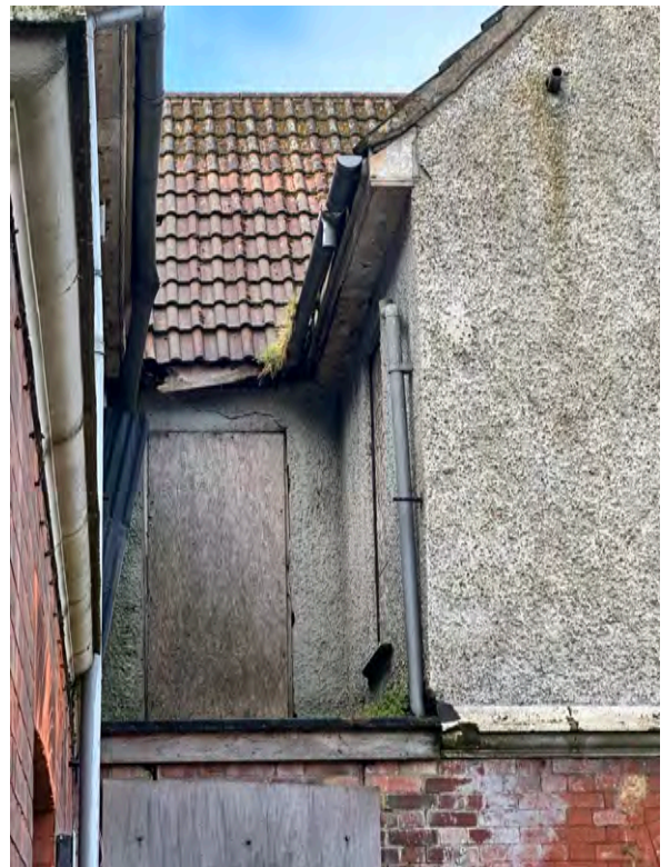
2.1.4.1 The gutters and down pipes are in poor condition, sections have failed and as such the discharge of rainwater is not being controlled and is therefore saturating the building fabric.
