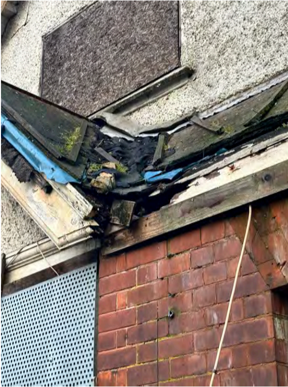
2.1.1.4 The flat roofs are felt covered, all are in poor condition.
