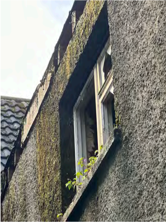
2.1.4.1 The gutters and down pipes are in poor condition, sections have failed and as such the discharge of rainwater is not being controlled and is therefore saturating the building fabric.
