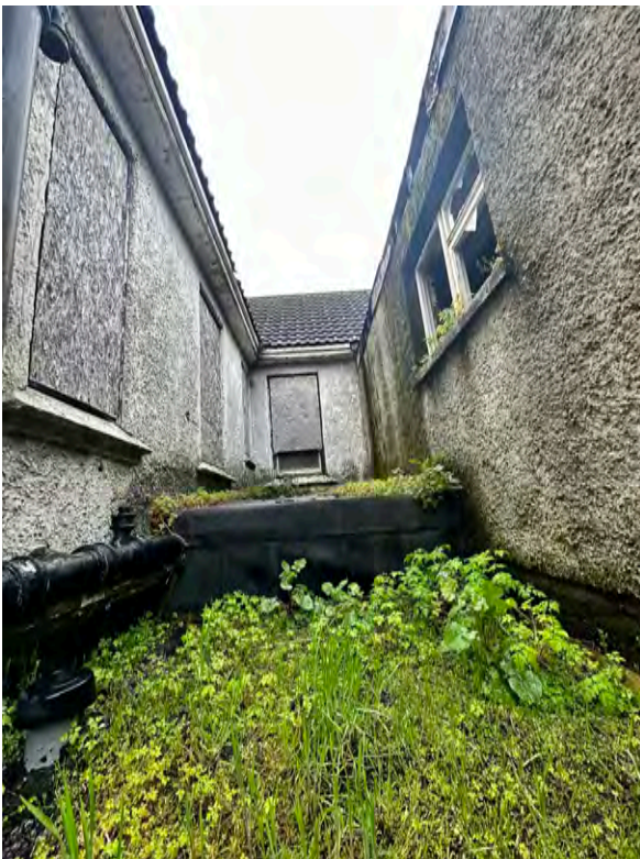
2.1.1.5 Over and above the immediate works to make safe the structure we recommend the roof structure be inspected prior to undertaking any replacement works to ensure the structure is capable to withstanding the proposed loads. Due to the age of the building the original roof coverings were most likely slate or clay plain tiles. Both of which are lighter than the replacement concrete interlocking tiles now fitted.
