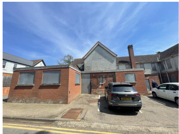
View of western aspect of B1
