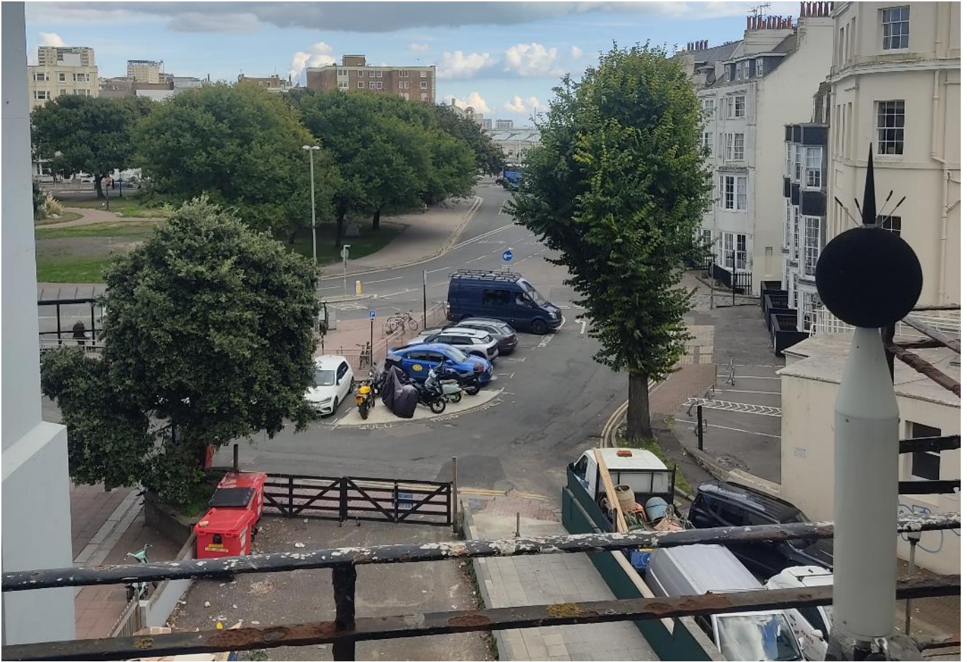
Location 2 – 1.5 metres above the 2 nd floor, looking east towards Old Steine
