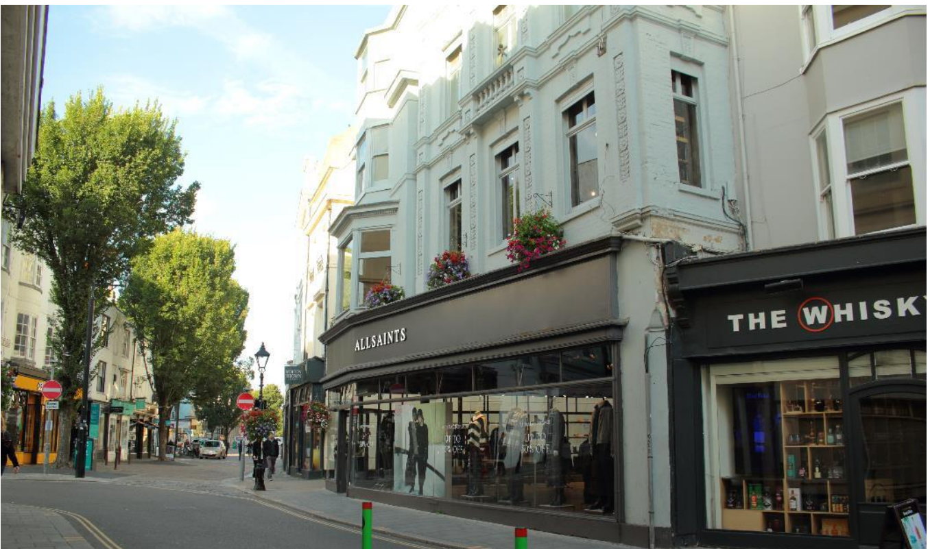
Looking north along East St at Location 1
