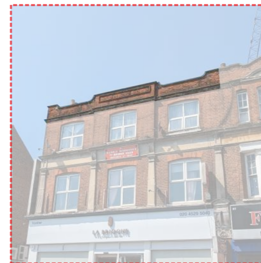
Figure 26 (left & middle): Example of C&Ps previous work to add an additional floor whilst successfully matching the existing brick work Figure 27 (right): Brick parapet detail retained in the proposed top floor terrace
