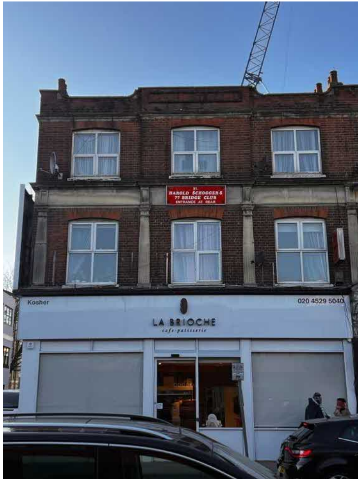
Plate 1: Overview of the building – eastern elevation
