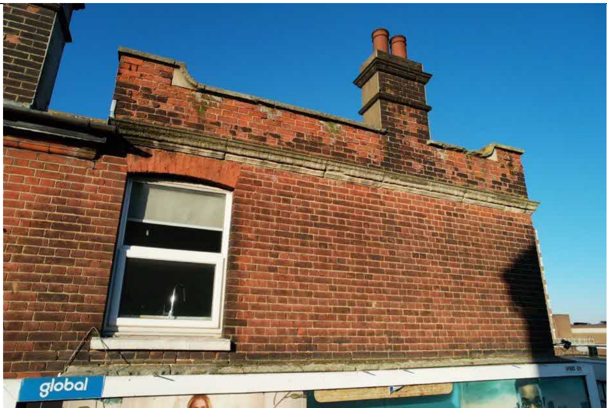
Plate 4: Southern elevation of the building
