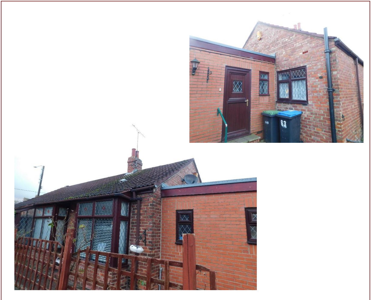
Figure 9 – General roof images
