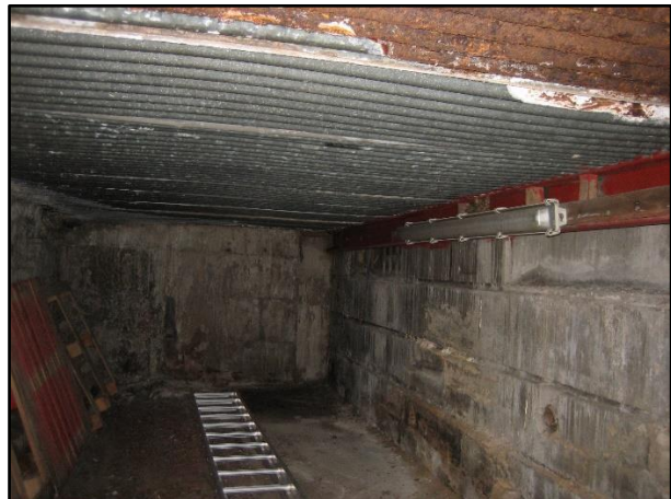
Area beneath projecting sales bay to front elevation
