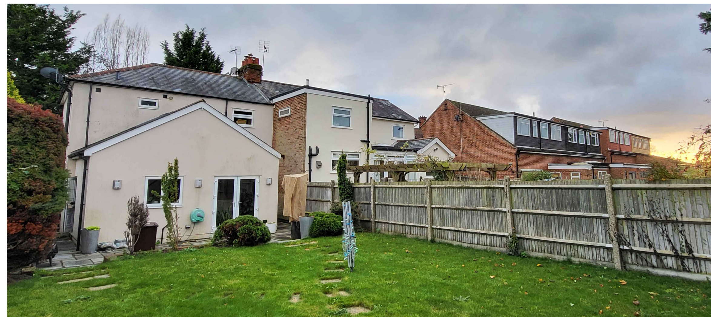
Rear View (including neighboring properties)
