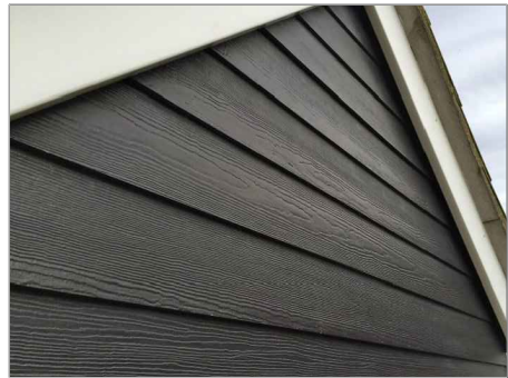
COMPOSITE SELF-COLOURED WEATHERBOARDING - FINAL COLOURS AS NOTED
