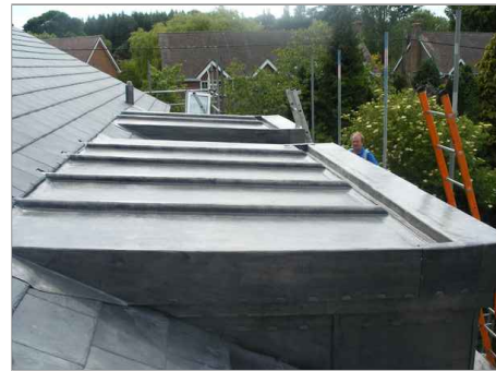
LEAD OR SIMULATED LEAD FLAT ROOF
