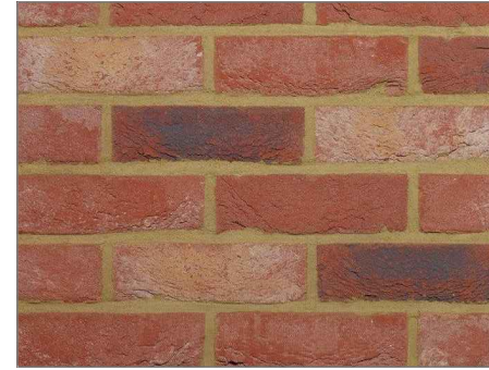
MALDEN ANTIQUE ESSEX RED, SEAFORD RED OR SIMILAR MULTI CLAY FACE BRICKWORK WHERE SHOWN
