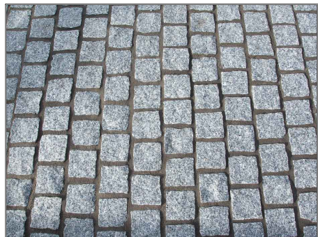
GRANITE SETTS - COBBLED DRIVEWAY ENTRANCE
