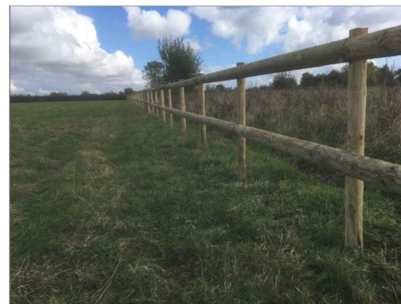
2 RAIL, HALF ROUND, POST AND RAIL FENCING TO SCREEN FRONT OF SITE
