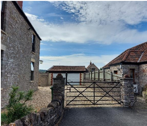
Figure 6.10: Garage to the rear of Close House on Upper Tockington Road
