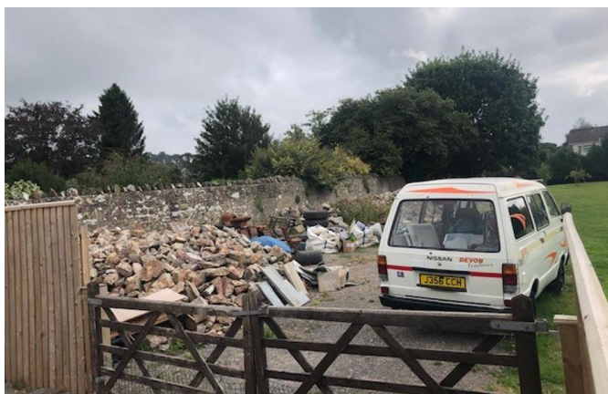
Image 8 – Rear garden and access to new dwelling and garage
