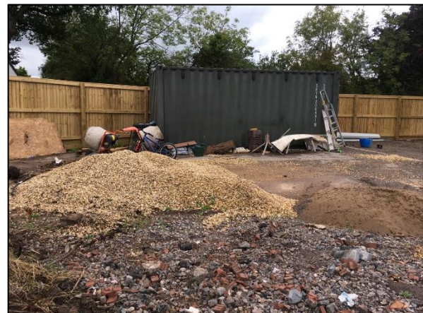
Photo 5 Vacant or derelict land
