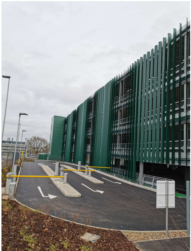
Figure 7 Car Park entrance to remain in place
