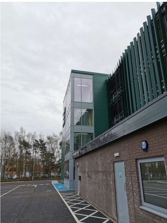
Figure 6 Stair core & Kiosk to remain in place.
