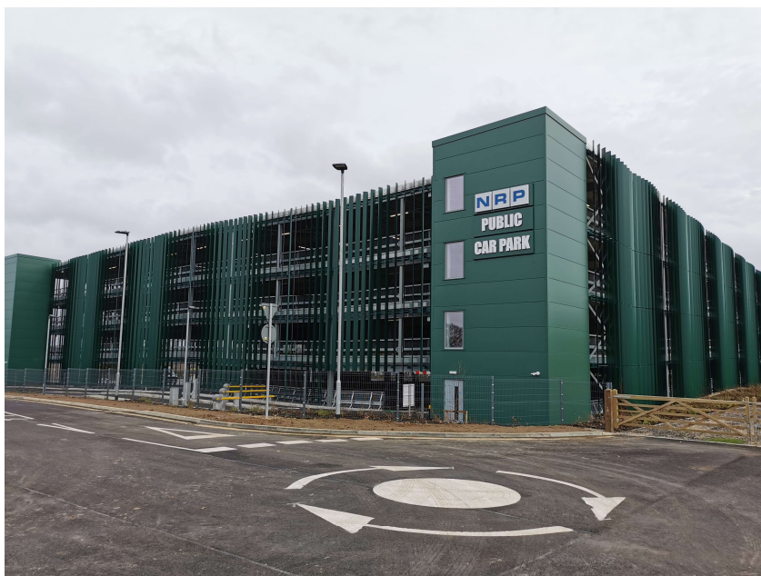
Figure 2 Existing MSCP - North West Elevation
