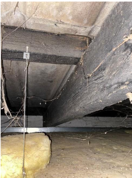
Internal views of loft space Fig. 13
