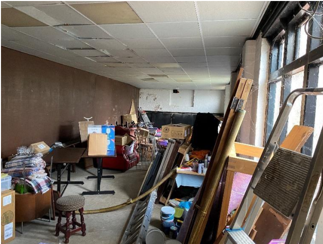
Fig. 11 Internal view of skittle alley towards the north.
