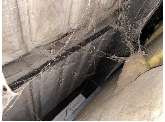
Fig. 12 Internal view of loft space
