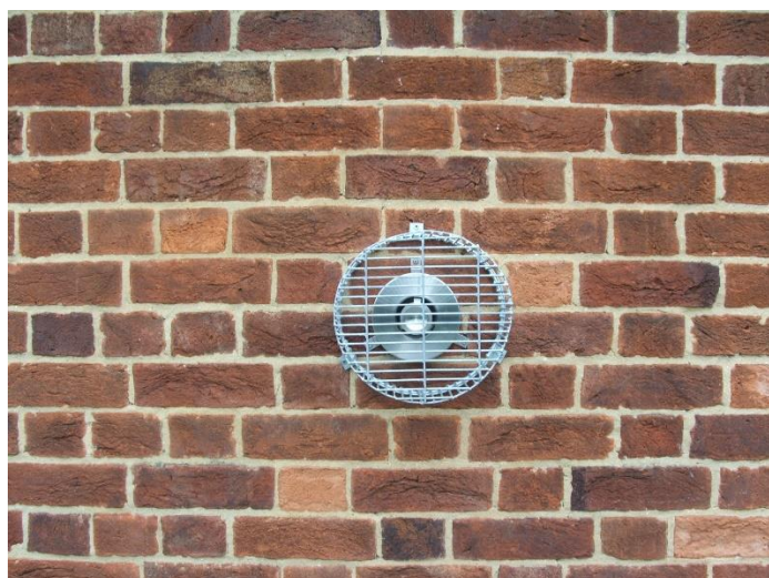
130mm diameter flue terminal with 24mm projection.
