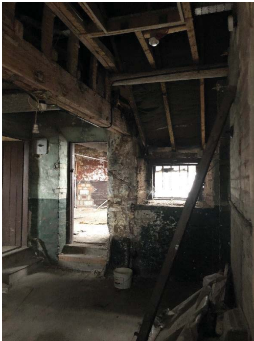
Figures 29 and 30: room at rear of the second floor, showing doorway to western room and condition of roof beams
