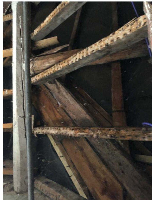
Figures 33-34: Western room on second floor, collapsed roof beams and replacements and window detail
