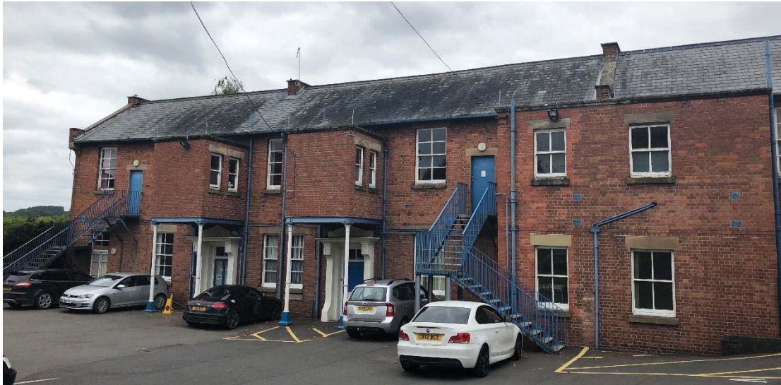
Figure 40: External view of the south-western infirmary building (disused maternity unit)
