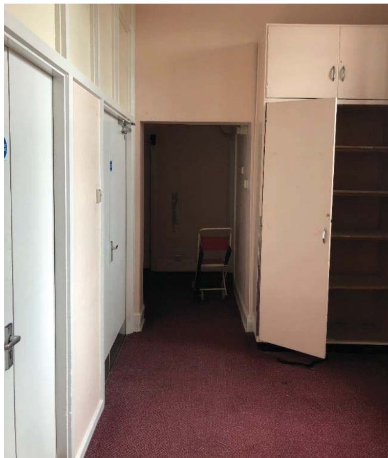
Figure 44: Corridor extending along the front of the building with wards off to rear
