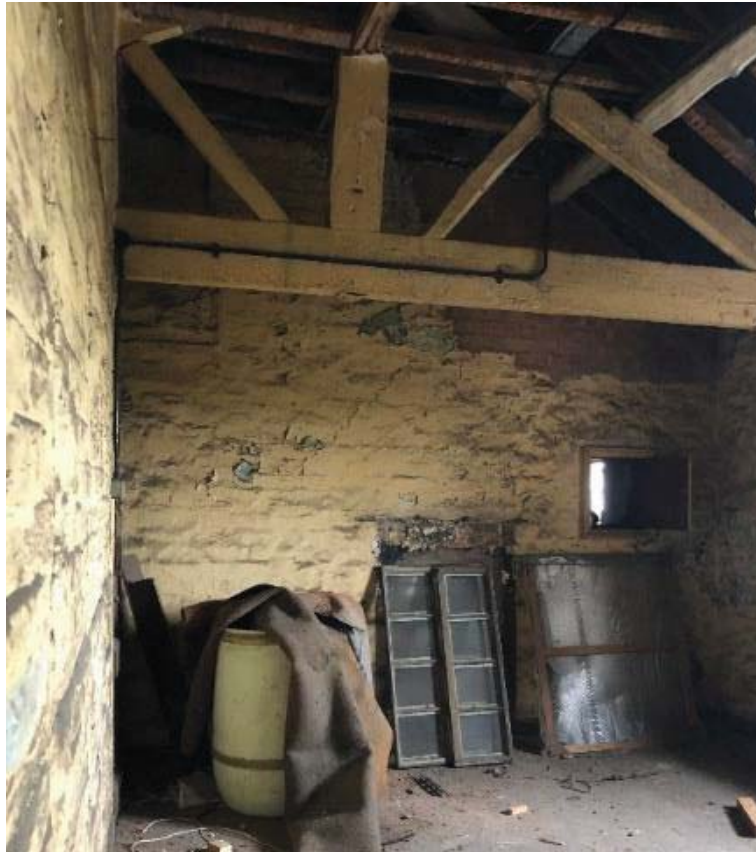
Figures 37 and 38: front central room of second floor (repaired roof structure)
