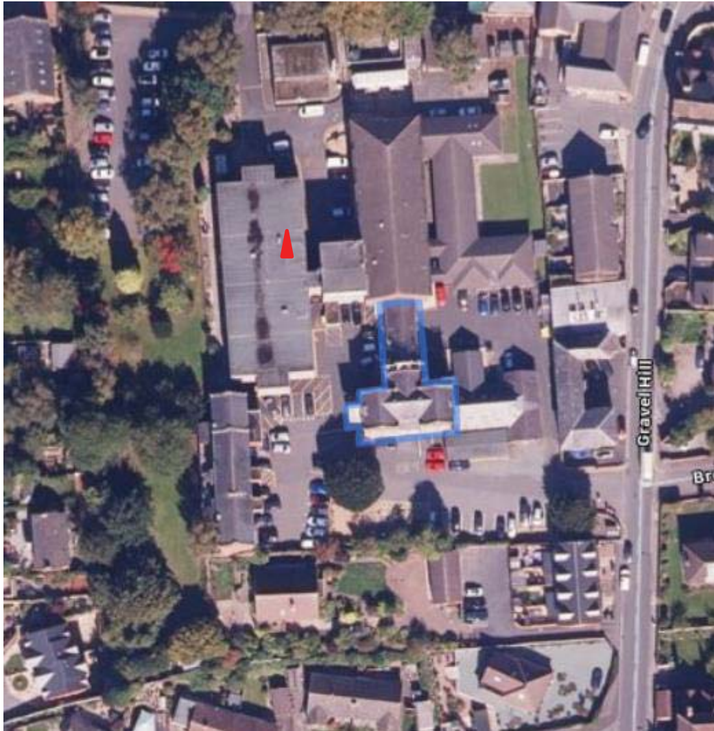
Figure 1: Aerial view showing the location of the main Grade II Listed Building at Ludlow Hospital. The red triangle indicates the position of the identifier on the listing map, the buildings are interconnected.
