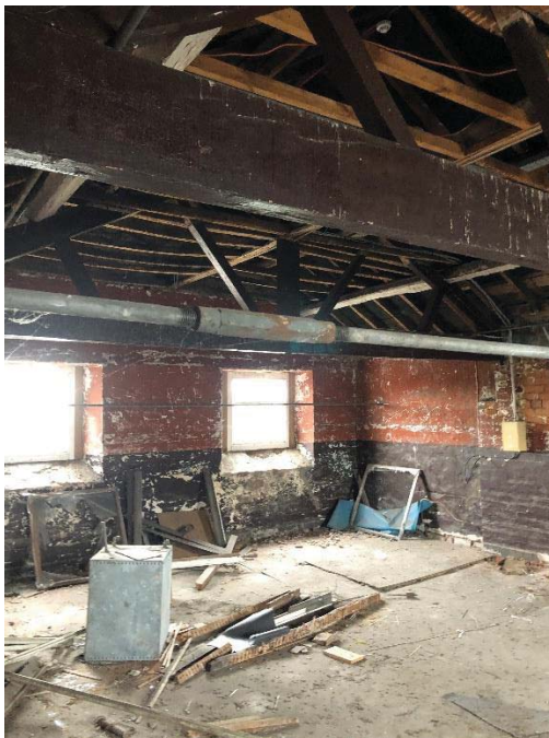
Figures 33-34: Western room on second floor, collapsed roof beams and replacements and window detail
