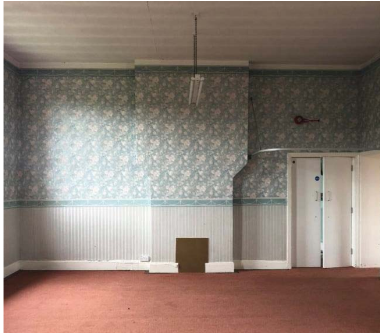
Figure 41: Example of the one of the larger second floor rooms
