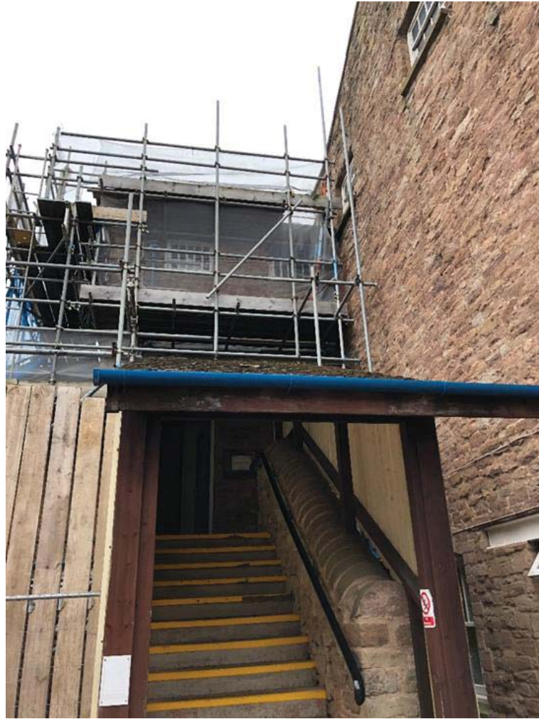
Figure 22: Stairway to the second floor of the entrance block
