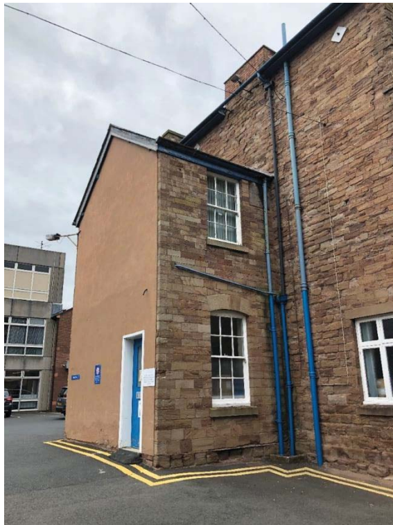
Figure 13: Western elevation of the entrance block, showing truncated western wing and brick chimney replacement
