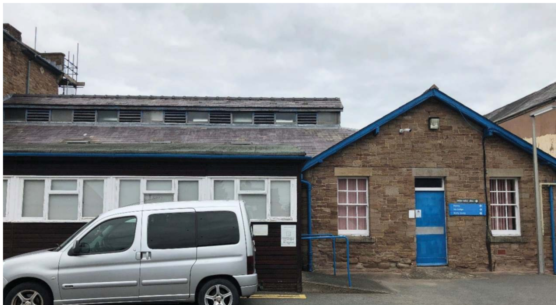
Figure 14: Vagrants infirmary (louvered clerestory roof visible), 1960s wooden shed at forefront, and range added prior to 1924 (right).
