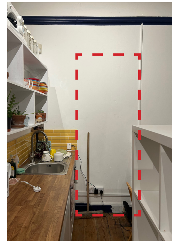
Unit 6 first floor opening located
