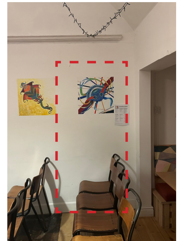
Unit 7 first floor opening located
