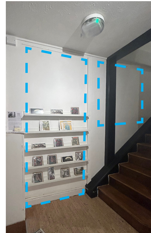
Unit 6 ground floor opening located
