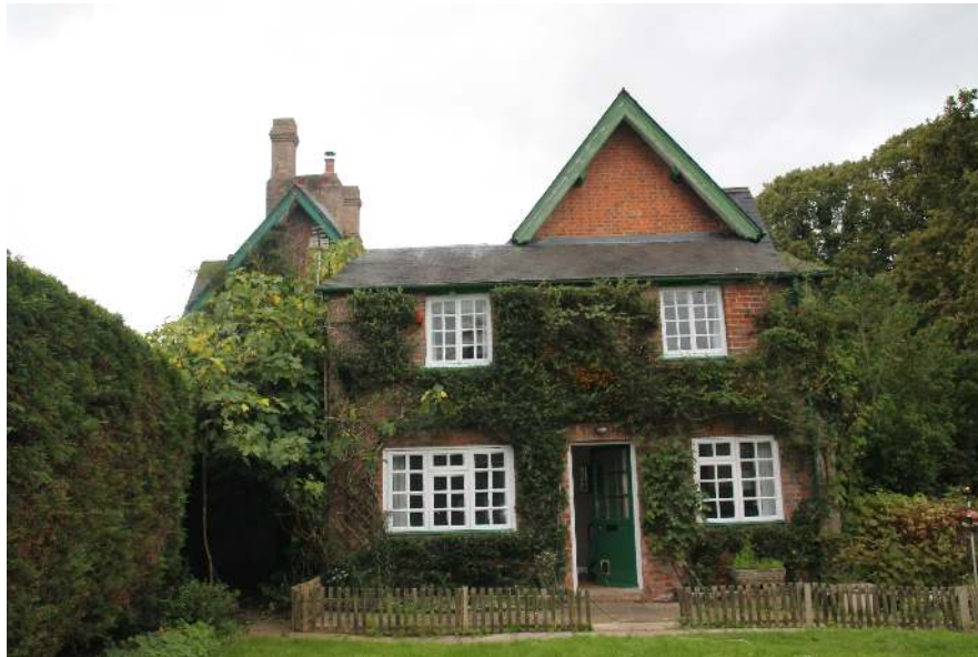
Fig. 10 (Above):- The rear range, which faces east, comprises small service rooms which has a monopitch slate roof. The service rooms are also a lower vertical scale to the rest of the building. There is also a change in material to red brick to the rear elevation of the building, which continues around the rear elevations of the two taller gables to the main building. This would suggest that the red brick is of less architectural significance than the buff bricks used on the main south, west and north facing elevations of the main house, and its use on the rear facing elevation of the building would mean it would have been out of sight. The windows to the north elevation are much simpler timber casement windows, of various ages.
