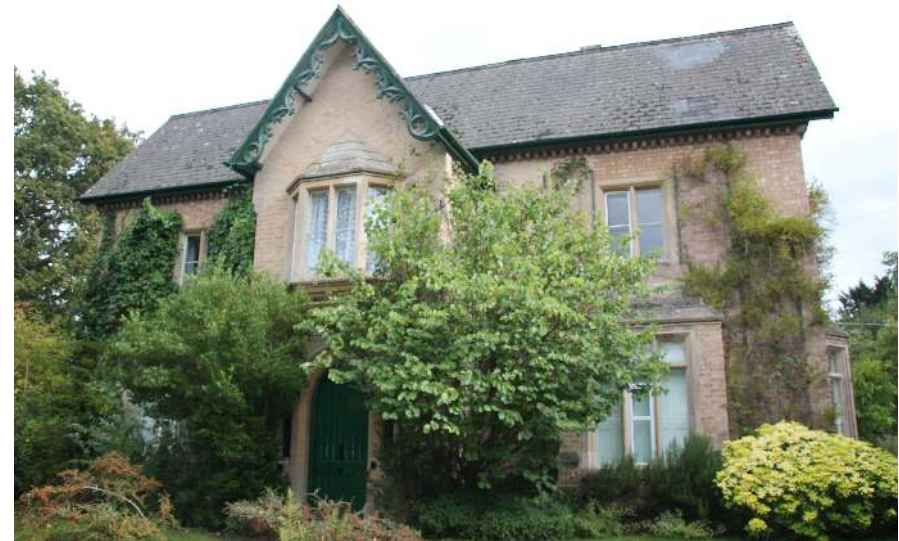
Fig 6 (Above): - West facing entrance elevation.
