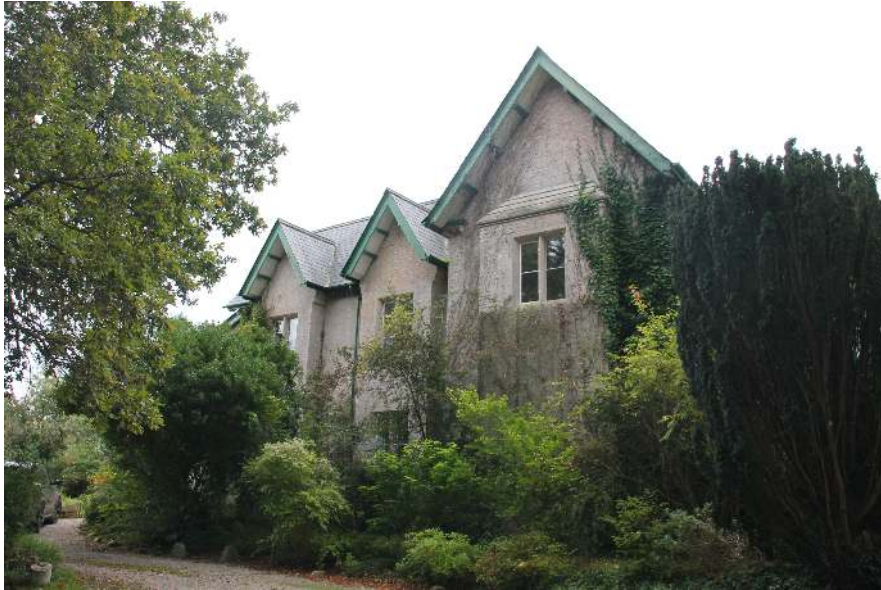
Fig. 8 (Above): - North elevation with projecting two storey bay window to the main range and two smaller gabled projecting bays. The gables have deep overhangs, with ornamental brickwork dentils between and stone surrounds to windows and stone corbels to the eaves.
