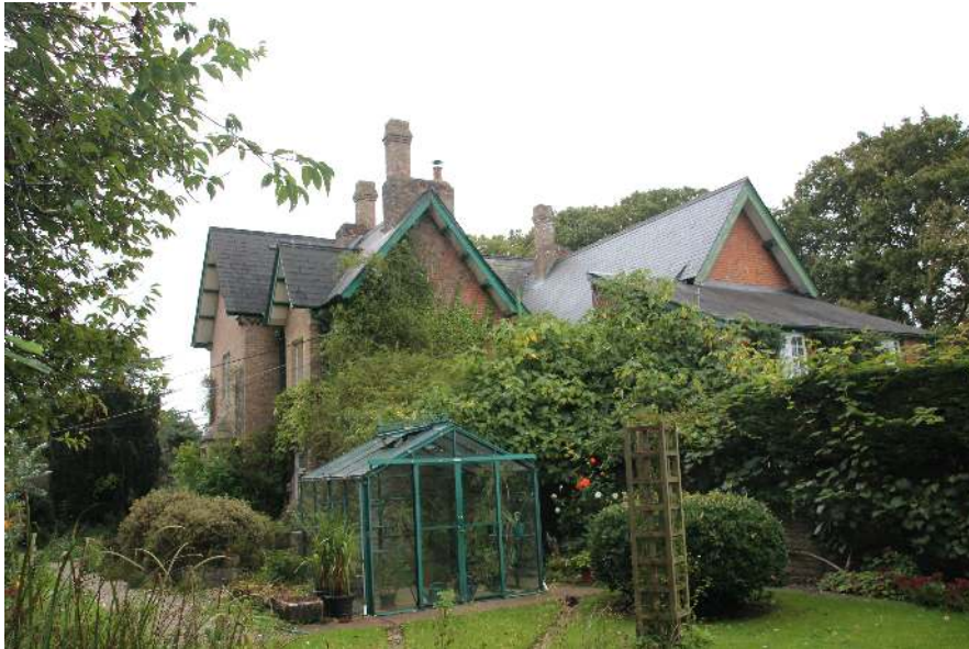
Fig. 11 also shows the chimneys having been truncated at some point since the engraving of the church, rectory and school was undertaken. The historic image shows each chimney with double stacks projecting from the roof, whereas they are now with only single stacks projecting from the original wider brick base penetrating the roof.
