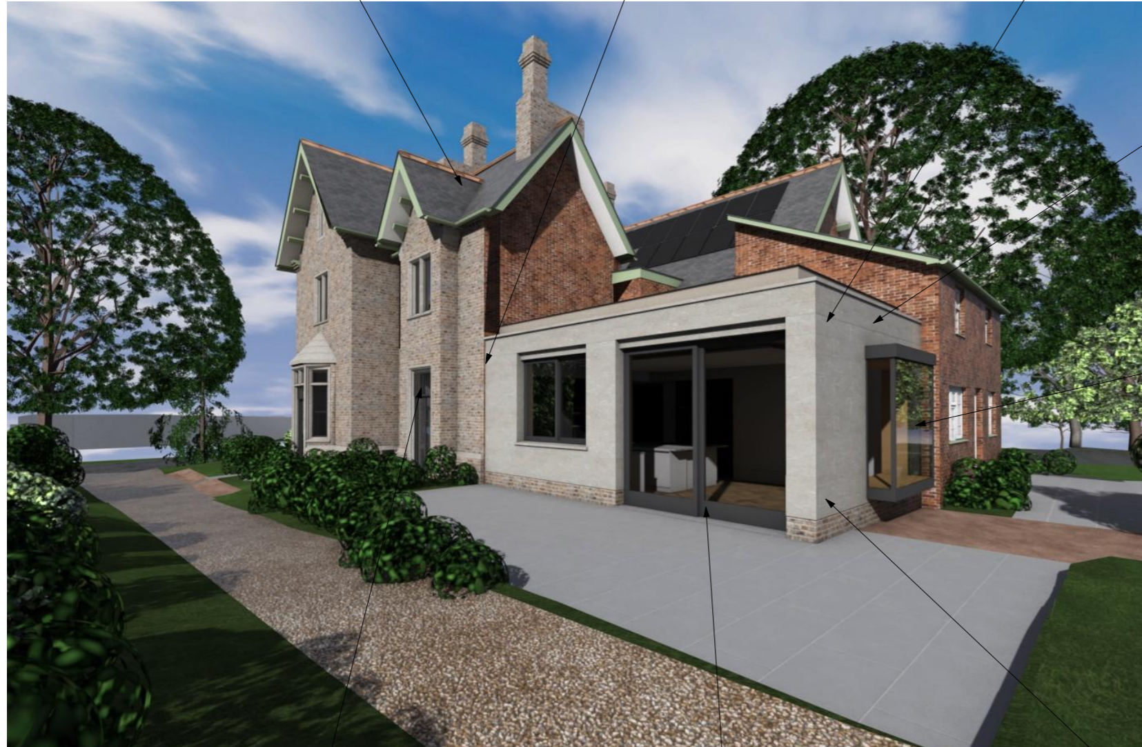
Replacement metal framed, 'crittall' style, glazed doors and windows to existing property
