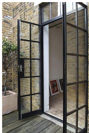
Replacement metal framed, 'crittall' style, glazed doors and windows to existing property
