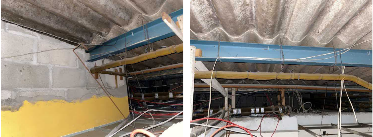
Figure 9: Example of the internals of the suspended ceilings in both buildings.
