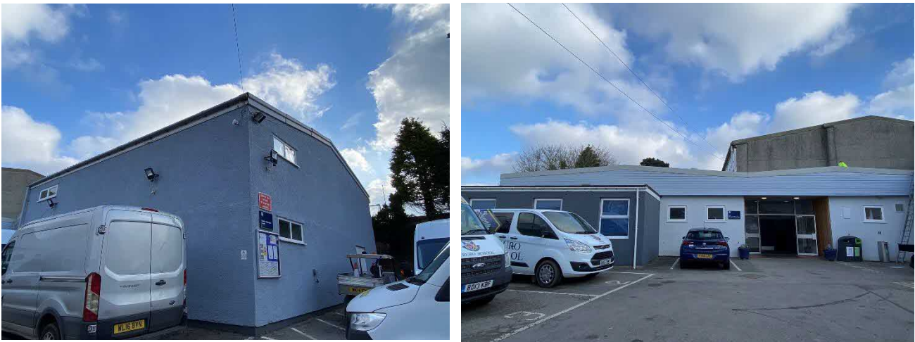
Figure 8: The externals of building 1 (left) from the south and building 2 (right) with small flat roof extension from the south.
