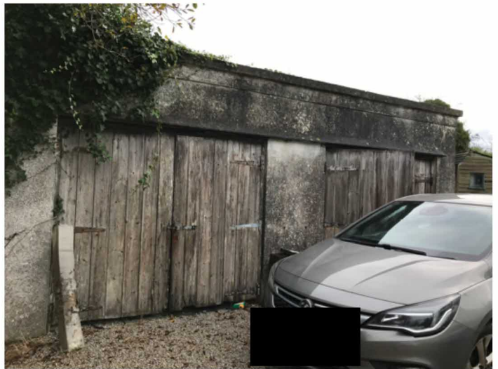
Image 9: External of garage
