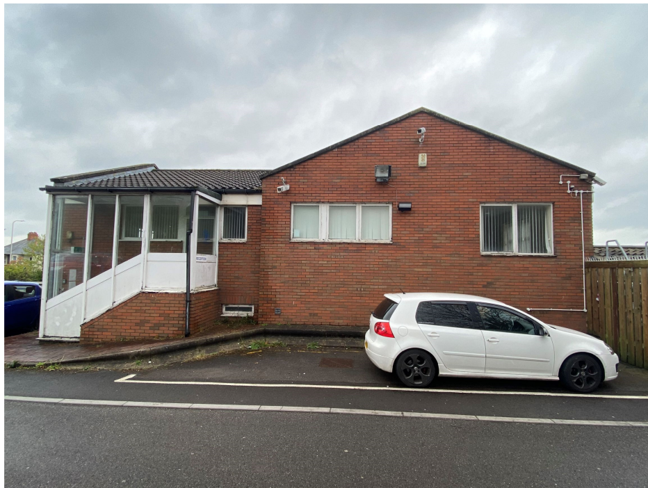
PHOTO 3 – OFFICE ENTRANCE NORTH ELEVATION
