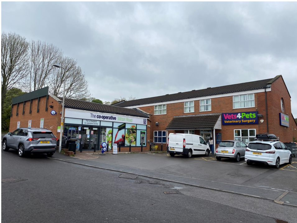
PHOTO 1 – BUILDING ELEVATION. OFFICES ARE FIRST FLOOR.
