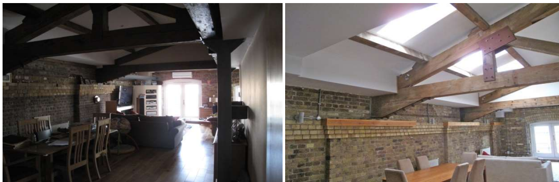
The image on the left shows the living room of Flat 120 on the 5 th floor and the image on the right shows the living room of a comparable flat on the 5 th floor with roof lights. The additional light enhances the warehouse features and reduces the requirement for electric lighting.
