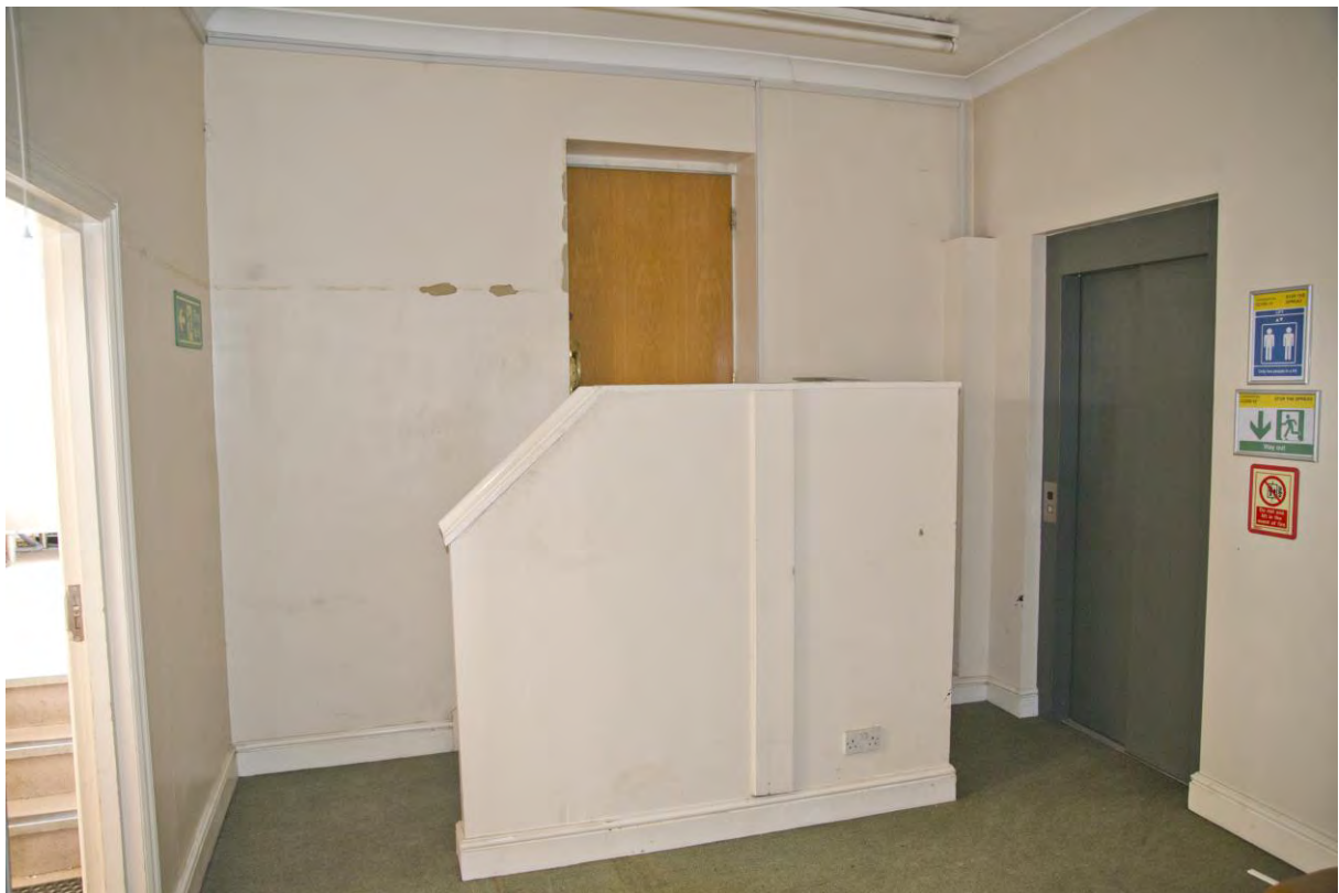
Plate 16 – No. 25 Queen's Road, first floor, southern circulation room. View looking south.
