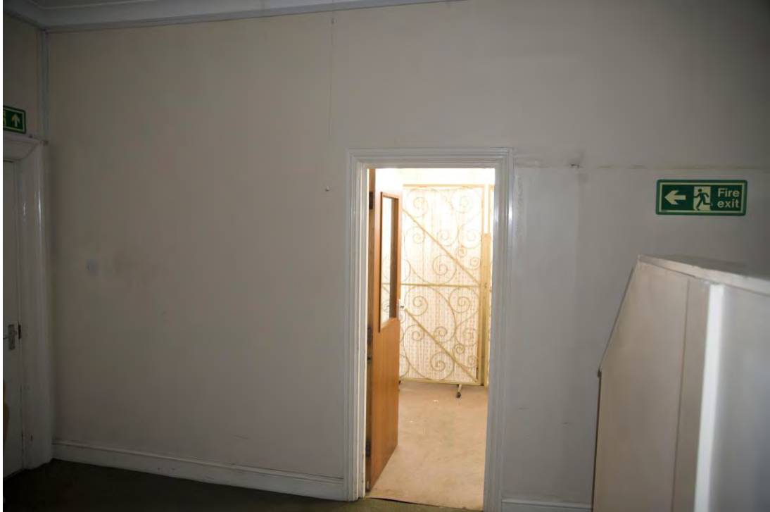
Suspected Phase 1 partition to the first floor of No. 25, south-western room
