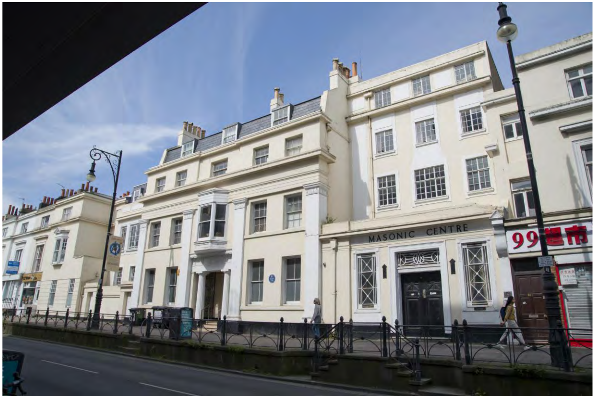
Plate 1 – The front elevation of the building, looking south-west.
