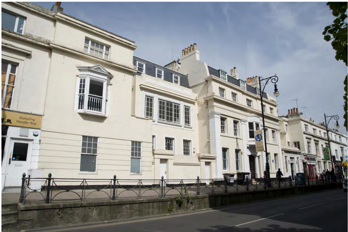
Plate 2 – The front elevation of the building, looking north-west.
