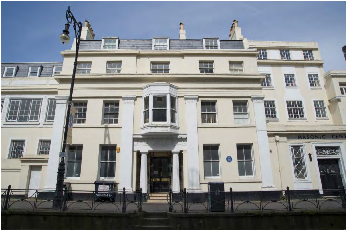
Plate 3 – The front elevation of No. 25, looking west.
