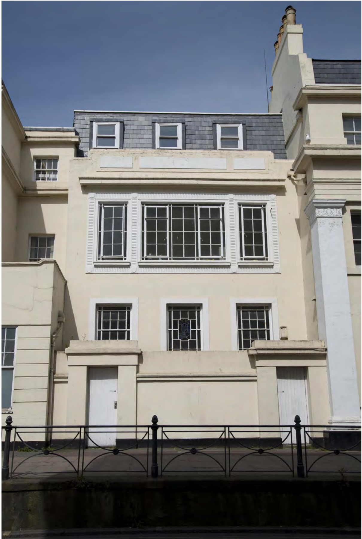
Plate 35 – Site of billiard room to the south of No. 25, front elevation looking west. Note Phase 1 garden wall with additional later gate.
