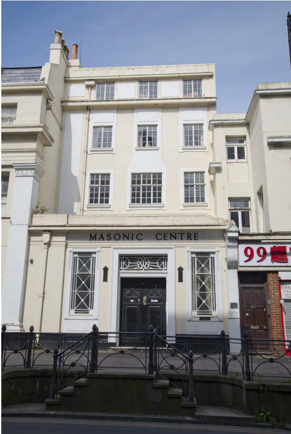
Plate 47 – No. 25 Queen's Road, Phase 3 entrance built on site of suspected Phase 1 service wing. View looking west.
