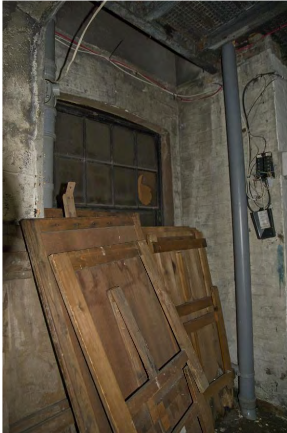
Plate 25 – No. 25 Queen’s Road, cellar, window to former rear lightwell, looking south-east.
