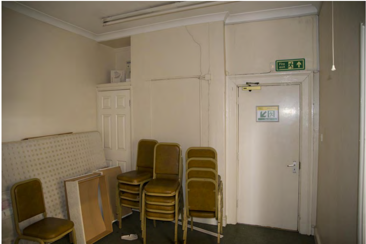
Plate 15 – No. 25 Queen's Road, first floor, southern circulation room. View looking north.
