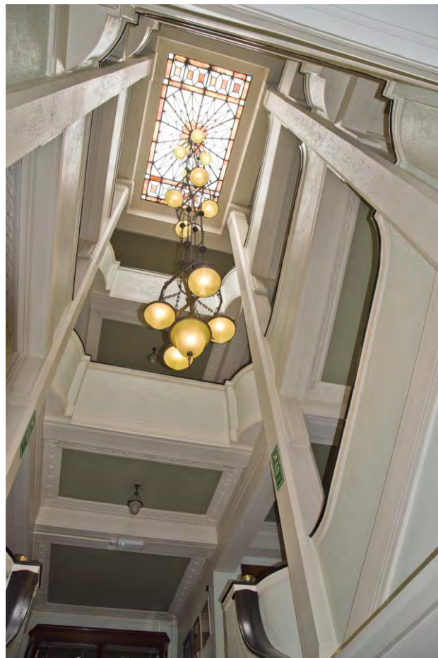
Plate 64 – No. 25 Queen's Road, Phase 3 main stairwell.
