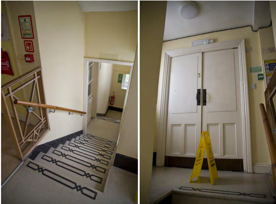
Stairs and doorway to rear corridor
