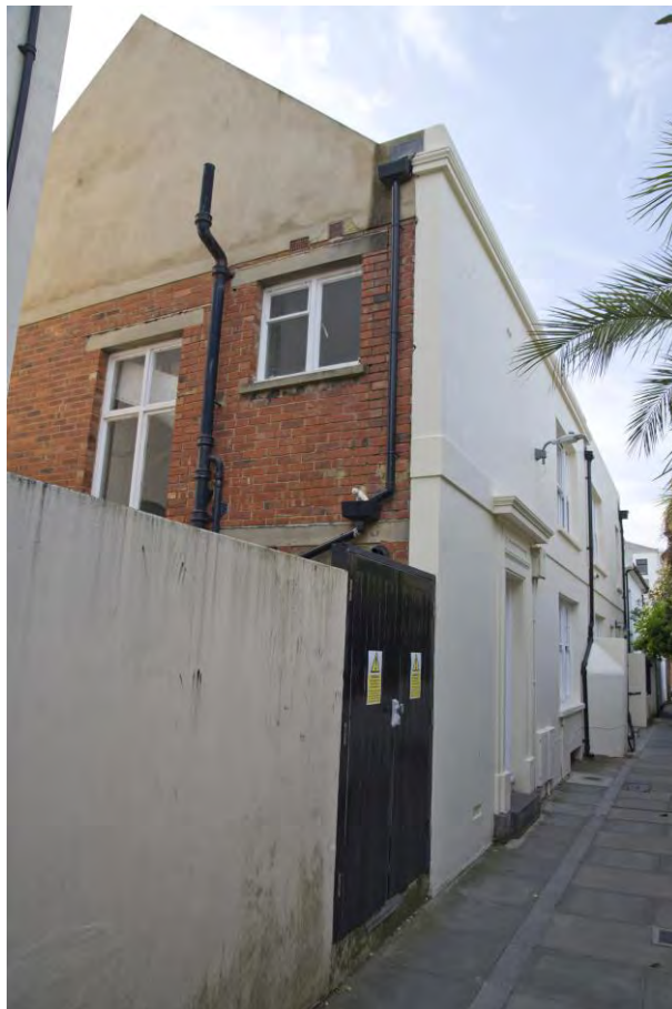
Crown Passage, site of proposed bin store entrance.
