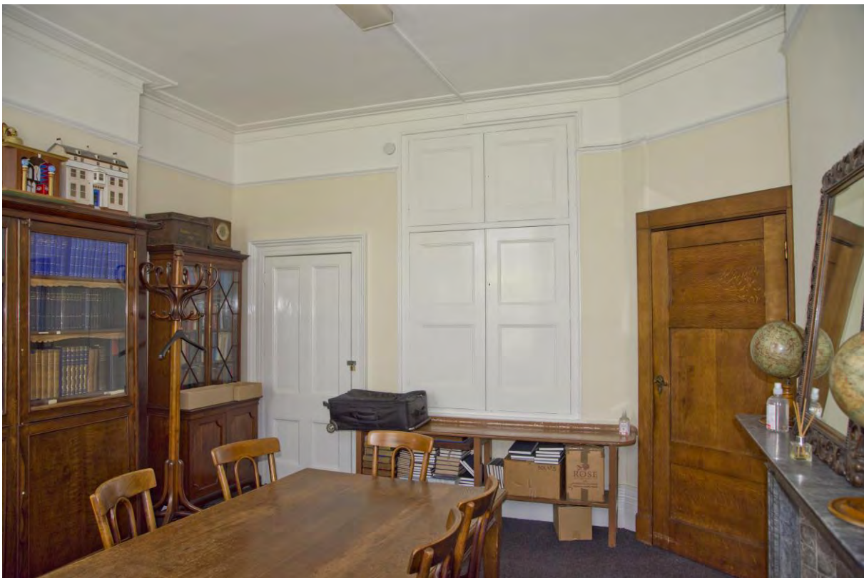
Plate 8 – No. 25 Queen’s Road, northern ground floor reception room, looking west. Note the inserted Phase 3 door.
