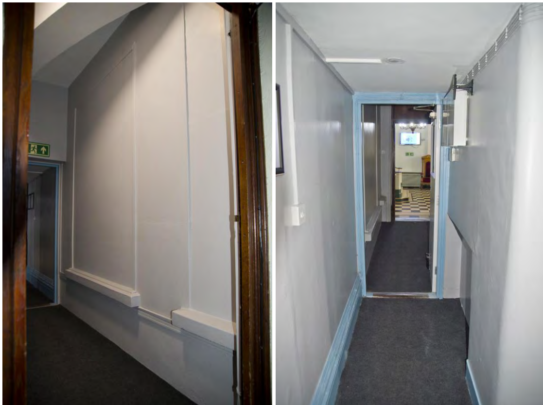
Plate 12 – No. 25 Queen's Road, ground floor Phase 1 service passage. Note blocked windows.
