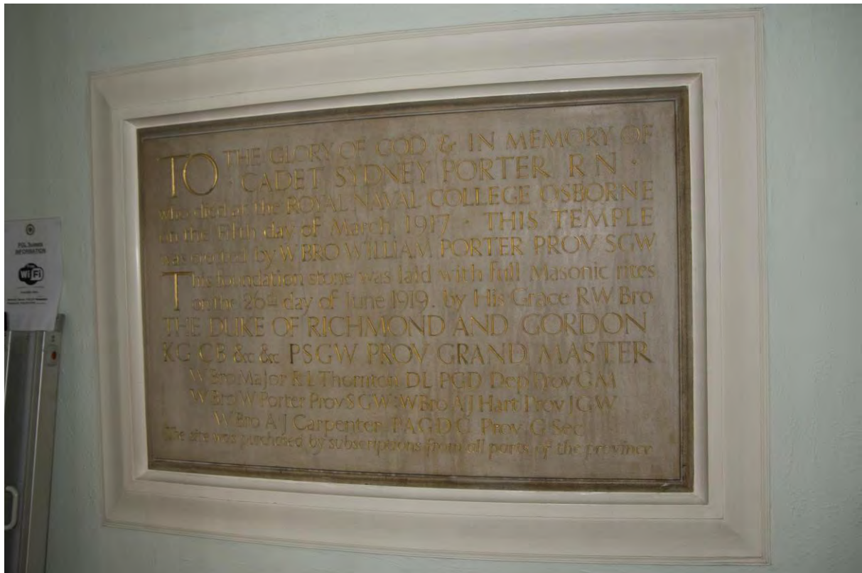
Plate 54 – No. 25 Queen's Road, foundation stone within Phase 3 ground floor entrance hall.
