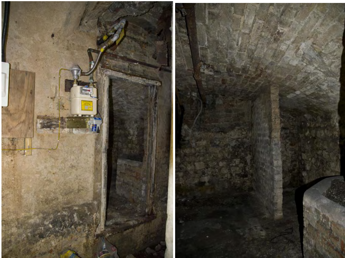
Plate 34 – No. 24 Queen's Road, former coal-hole in cellar.
