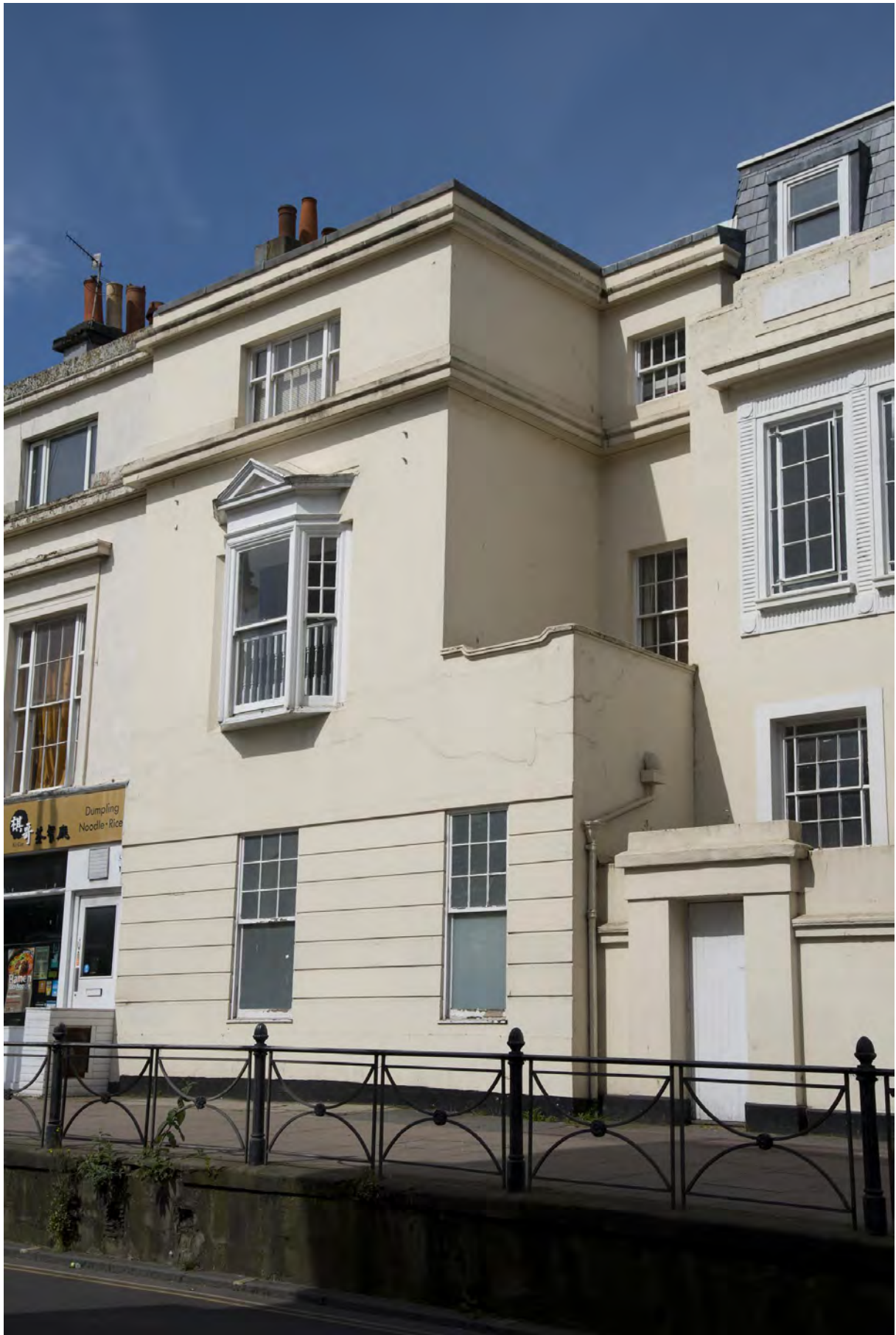
Plate 40 – No. 24, front elevation looking south-east.
