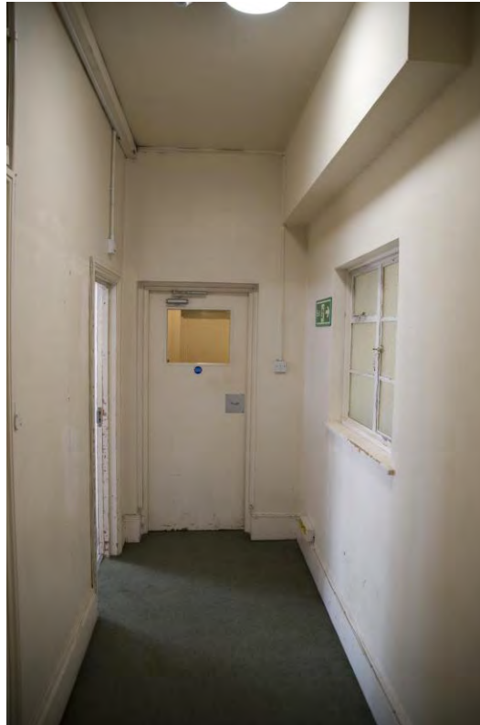
Circulation area to the north of the main Phase 1 stair at first-floor level
