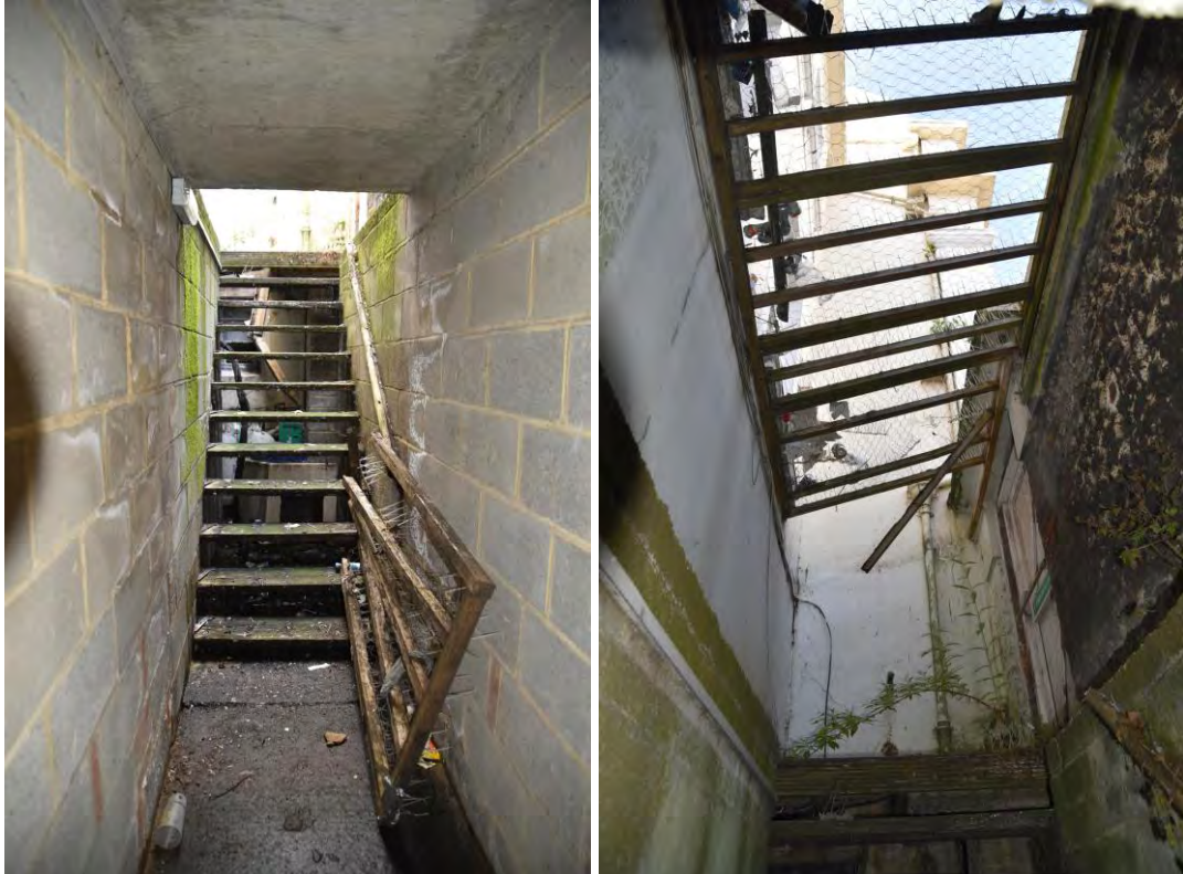
Front lightwell to the southern side of No. 25
