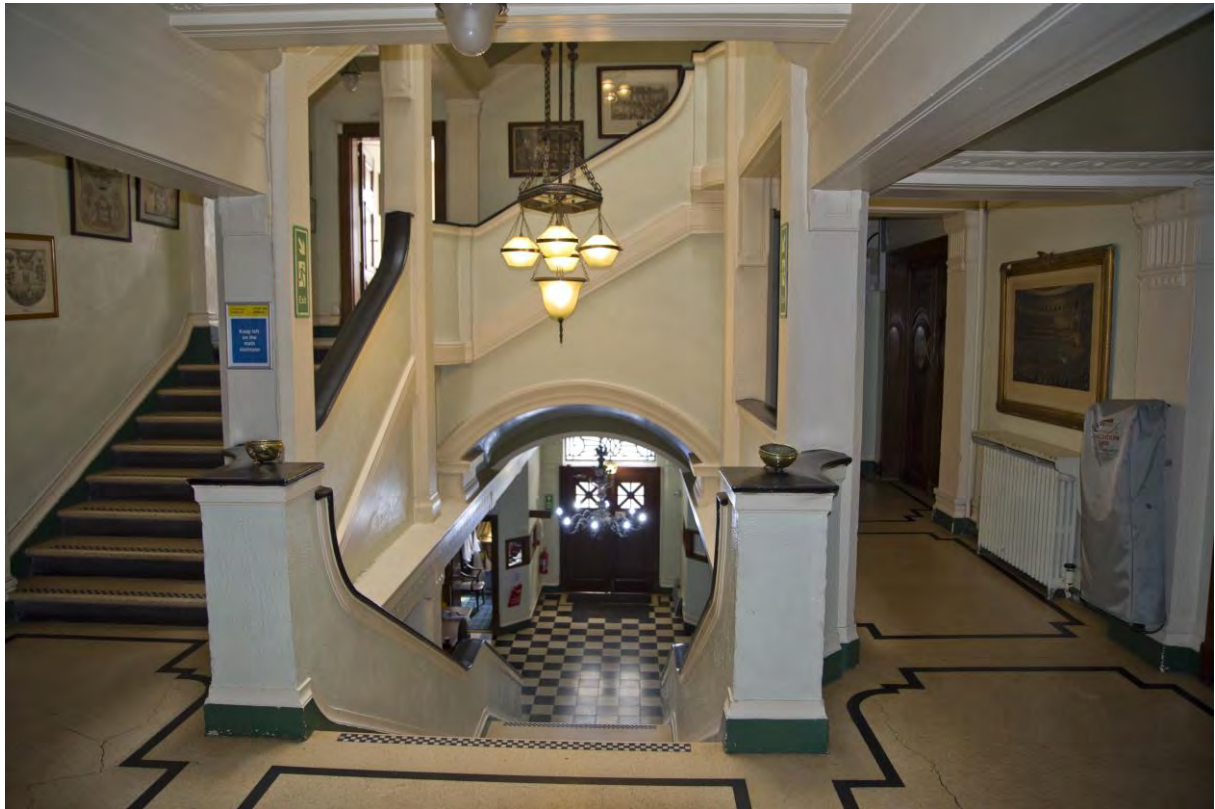
Plate 63 – No. 25 Queen's Road, Phase 3 stair and first floor circulation area. View looking east.
