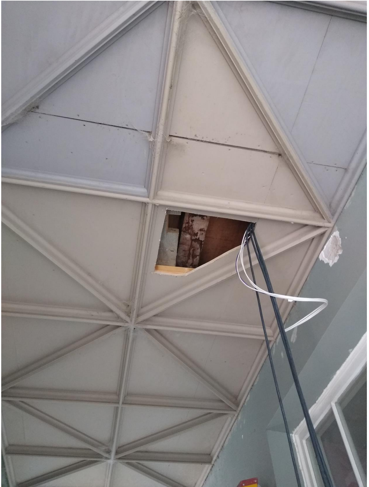
View of Existing External Soffit
