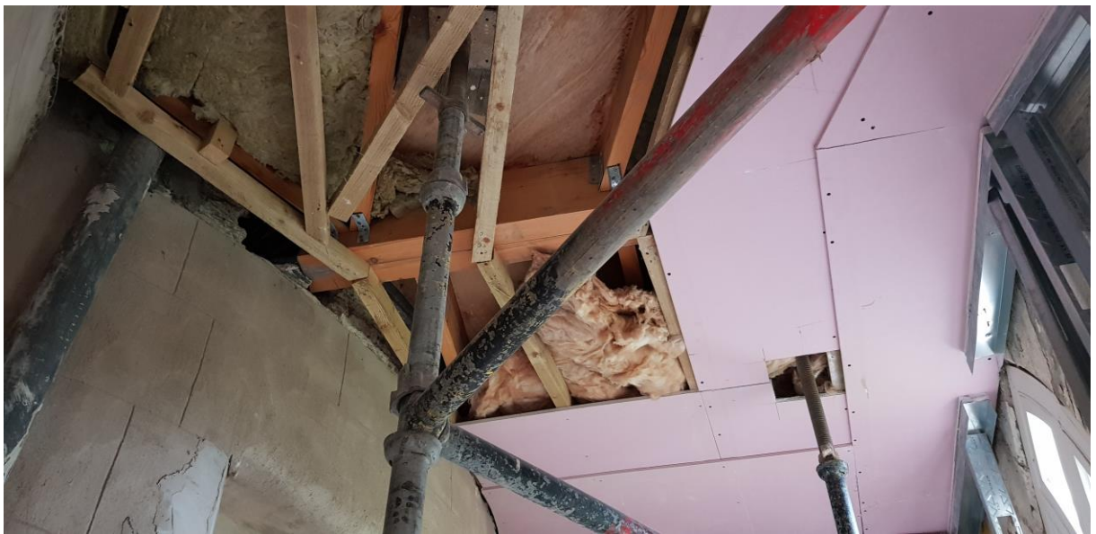
View of Existing Internal Soffit
