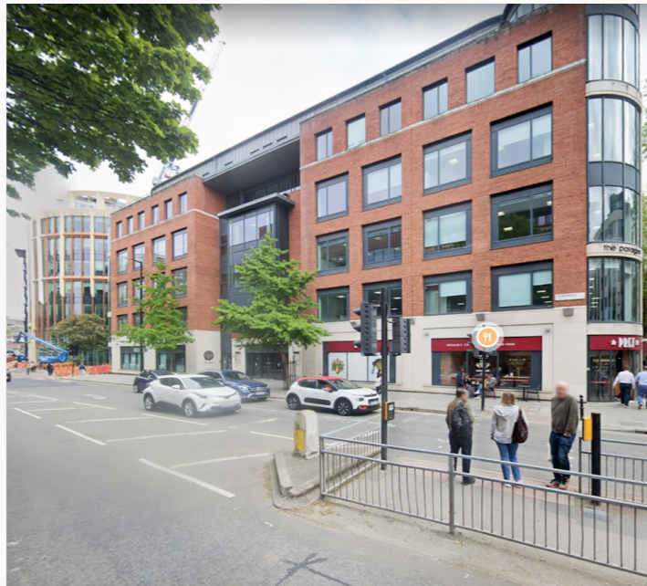
A - Victoria Street view
