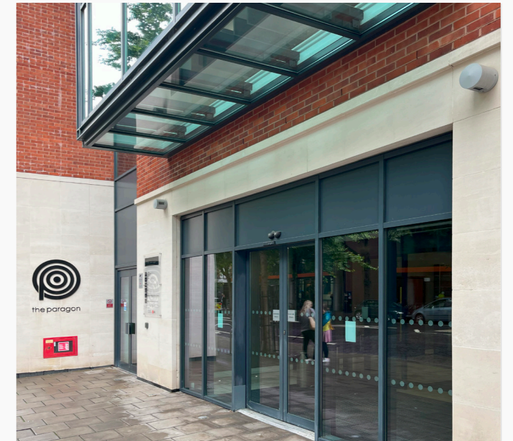
C - Entrance door
