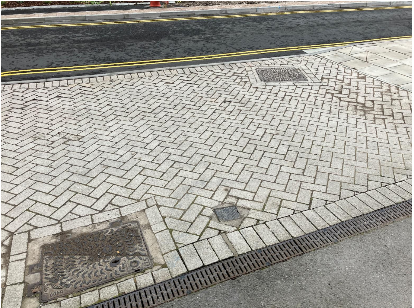
Figure 6: Showing surface water drainage on sidewalk
