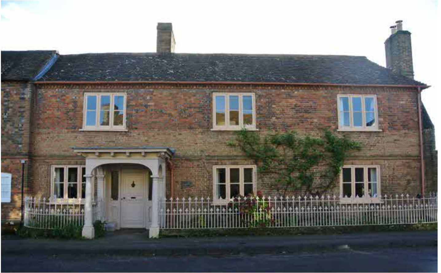
Front (west) elevation with 18th century entrance porch and 20th century casements
