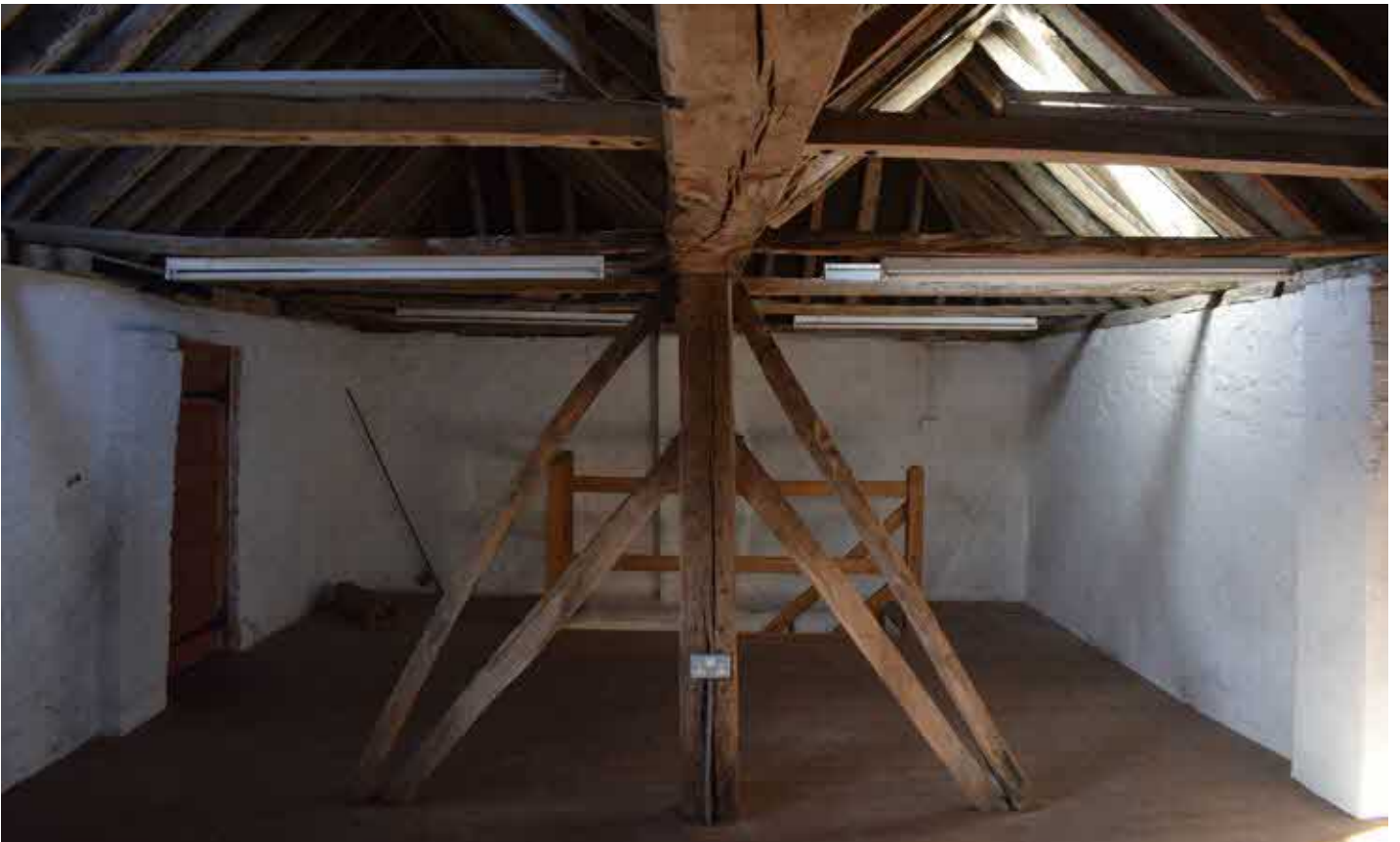
Upper level with later supporting column and bracing.
