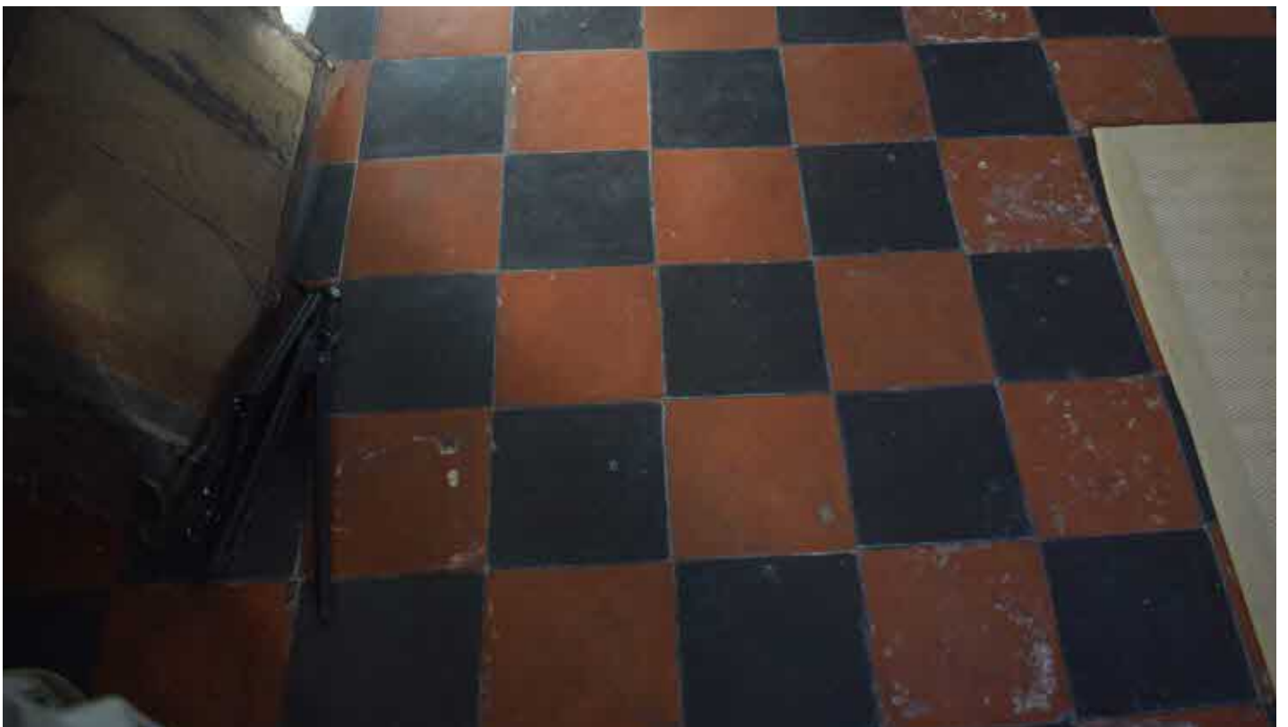
Large terracotta floor tiles to rear ancillary range
