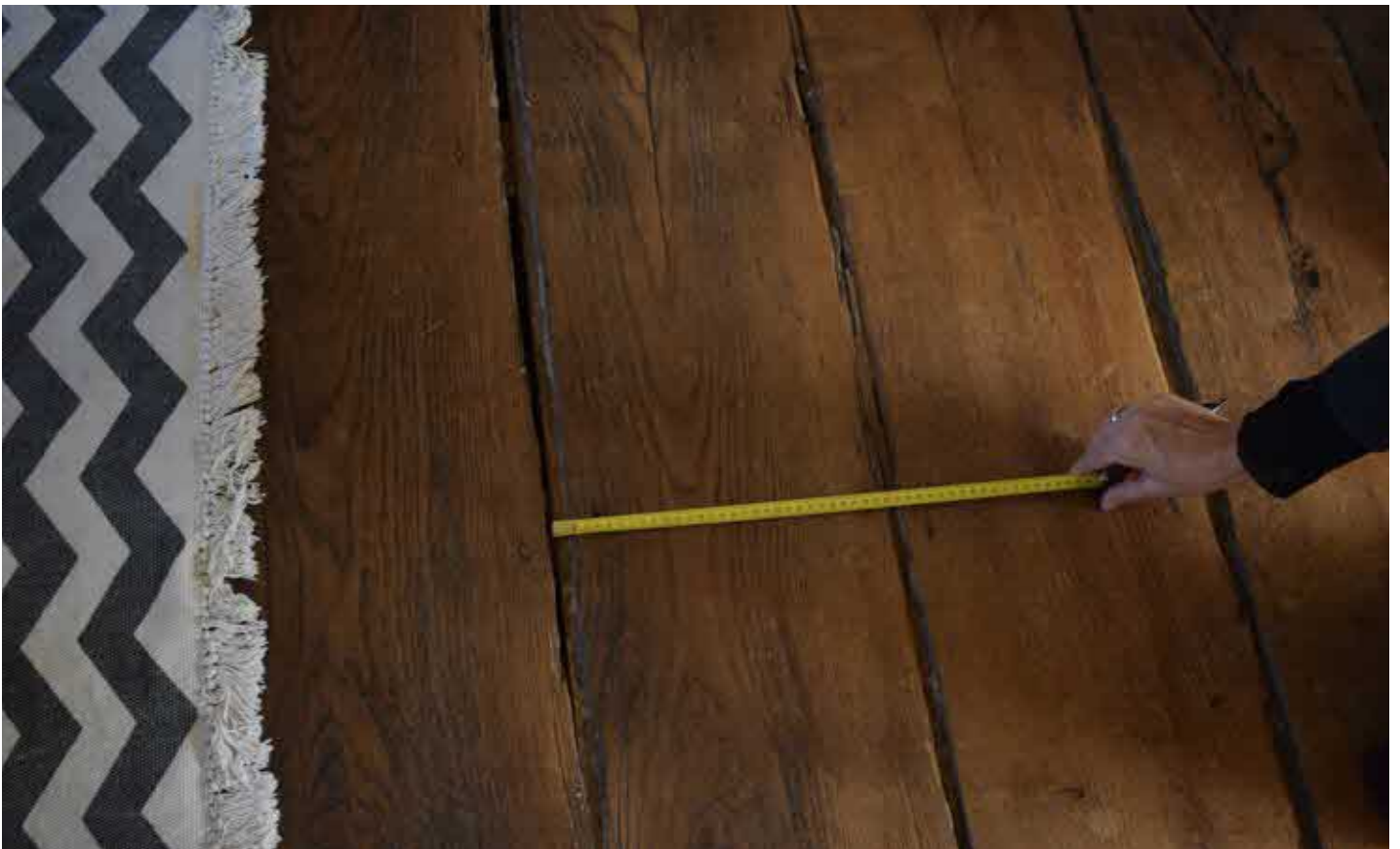
Wide floorboards (300mm) visible in one of the first floor rooms, as well as in the ground floor sitting room, suggest a late 17th early 18th century date.
