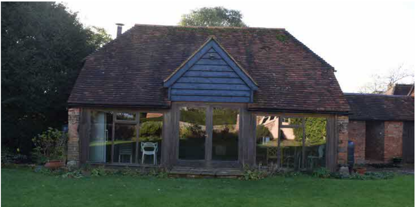
Garden elevation of barn/cartshed, with central timber gable, glazed doors under and glazed infill either side.
