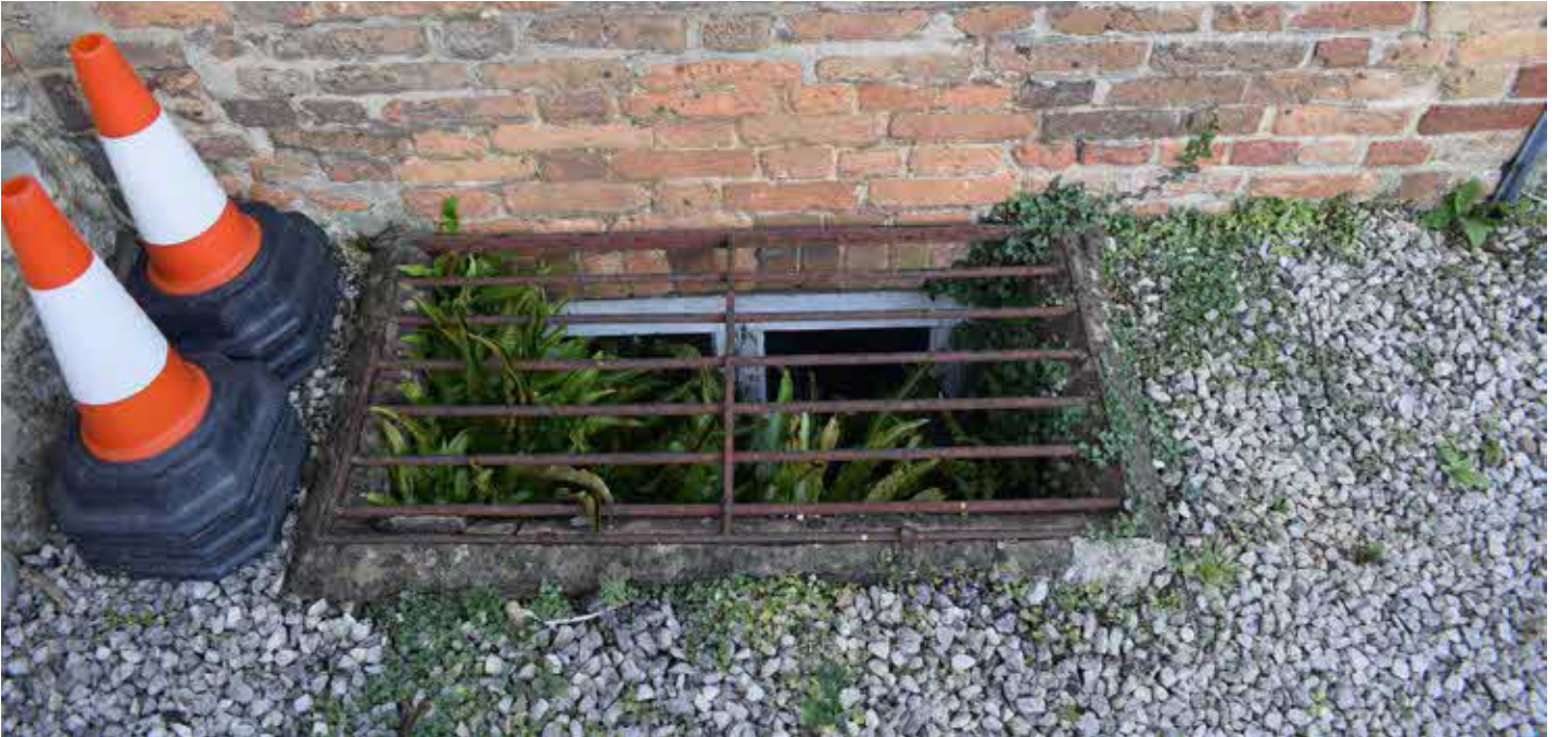
Cellar window protected by ground level grill.
