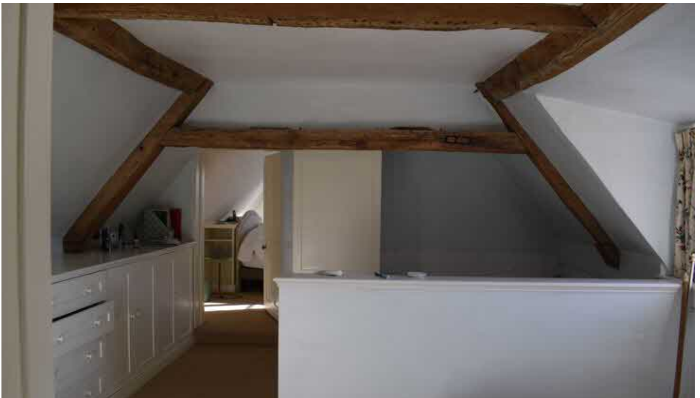
The first floor of the rear ancillary range has been inserted, possibly when the rear portion of this range was built. Timber framing visible is of a fairly basic quality, reflecting the earlier function of some form of double height agricultural building. Evidence from empty mortices and pegs remaining to principal rafter that the lower collar has been removed, probably when the floor was inserted.
