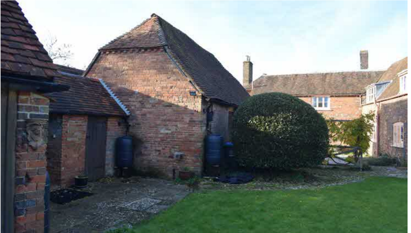
Rear wall of garage with linking shed to right.
