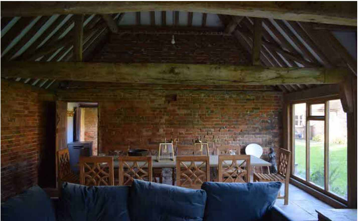
The barn has been recently converted (2005 LBC ref: 05/00436/APP) to form entertaining space. Timber queen post or strut roof trusses with purlin and rafters exposed.
