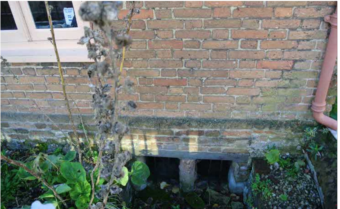
Stone mullioned cellar window in Front (West) elevation
