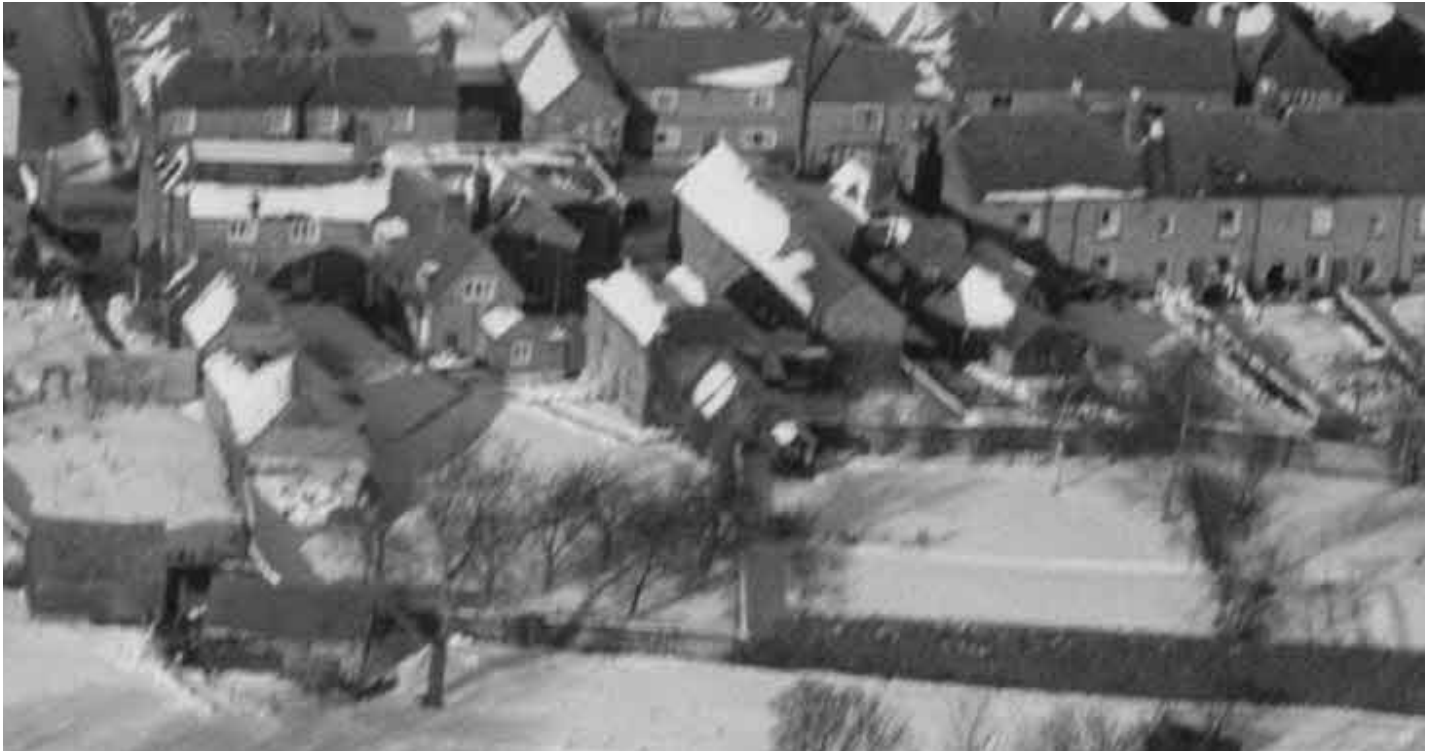
View from the south of 2 Temple Street, ranges of outbuilding to the rear, and the garden to the south-east (EAW047950 ENGLAND (1952). The village in the snow, Brill, from the south, 1952)
