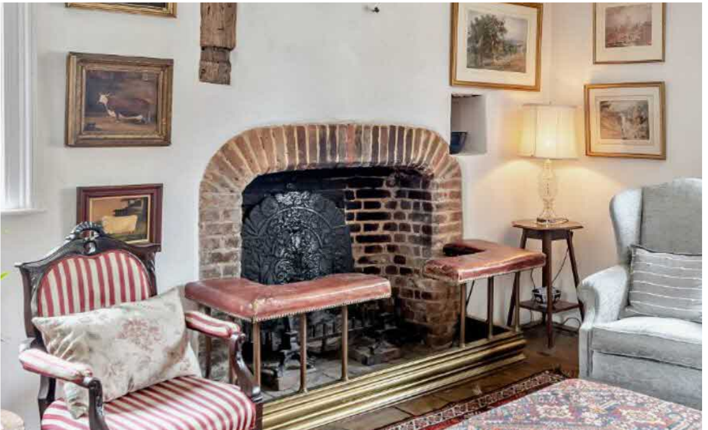
Brick arched fireplace to the southern chimneystack appears to be contemporary with the cellar and represents the oldest part of the house.
