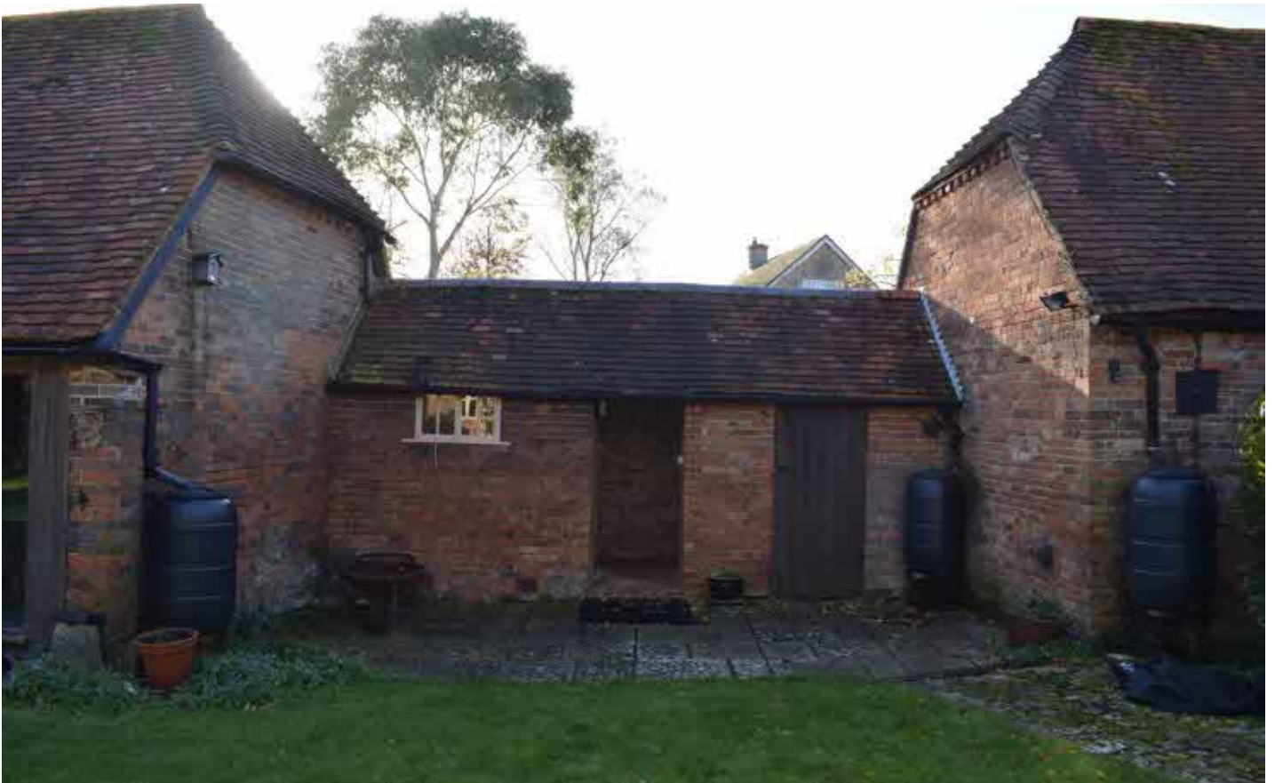
Linking single storey structure with shed to RHS, "Thunderboxes" area to LHS. Simple two light casement window.
