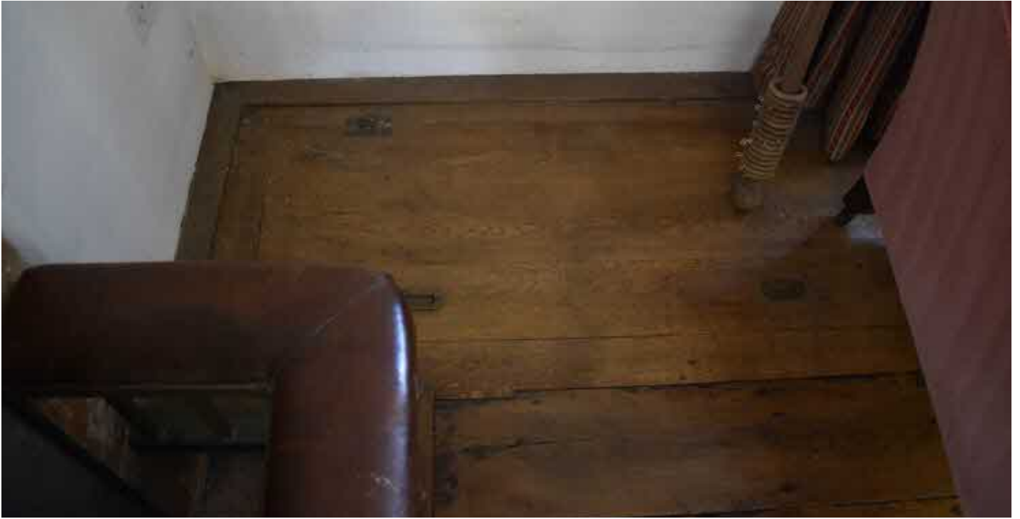
Trapdoor (now heavily restored) adjacent to fireplace gives direct access to the cellar below and references the previous commercial use of a bakery.
