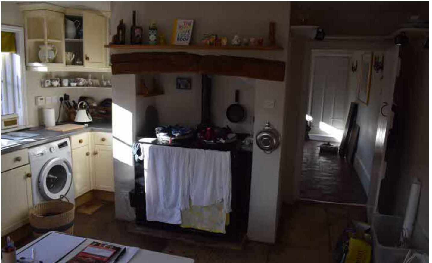
Fireplace in rear ancillary range kitchen. Non-original bressummer over fireplace and stone flags well set.
