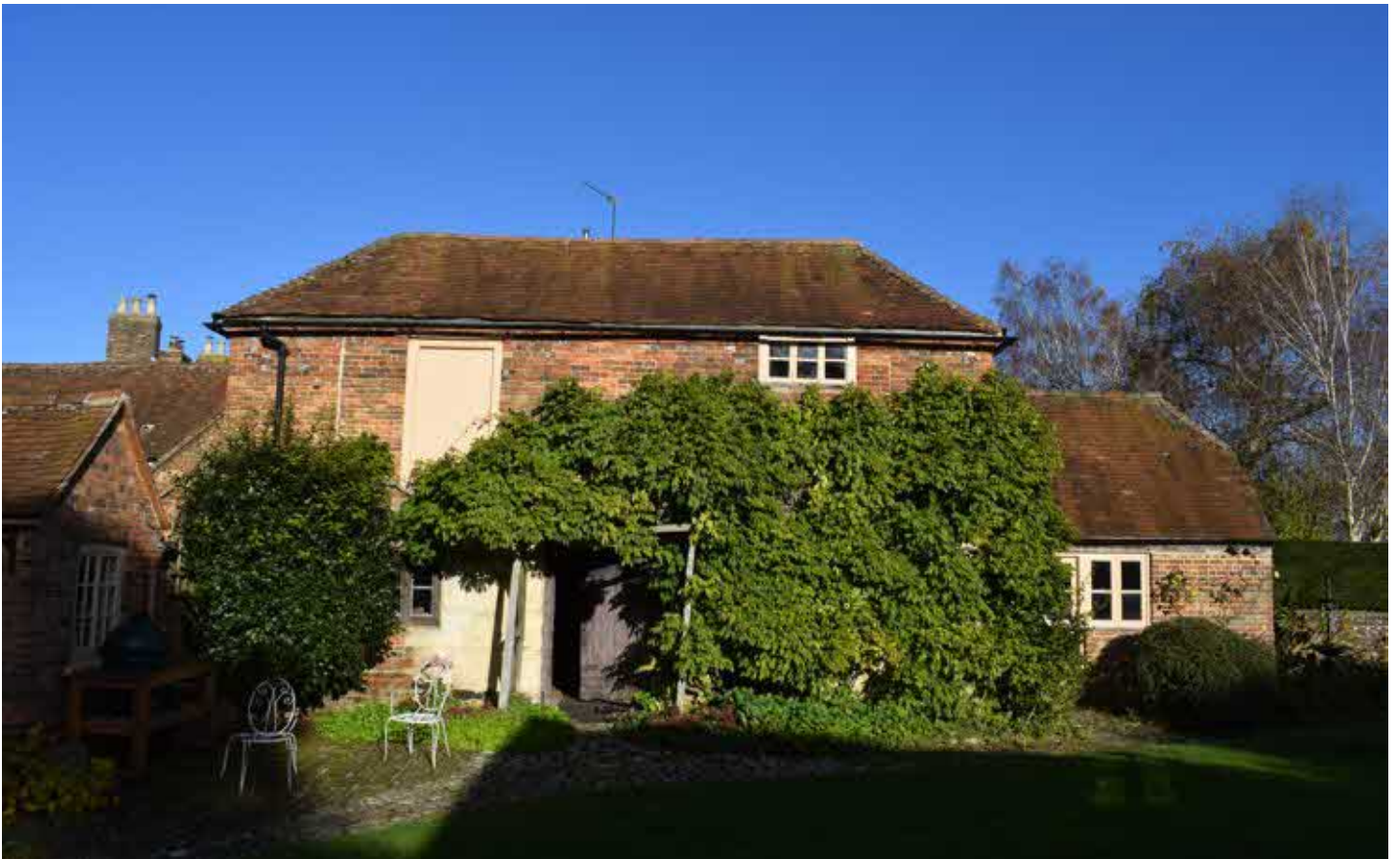
Stable front elevation with studio to RHS
