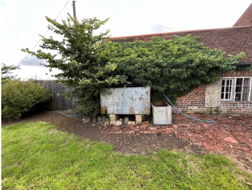
Climbers over roof, adjacent saplings, and tanks.
