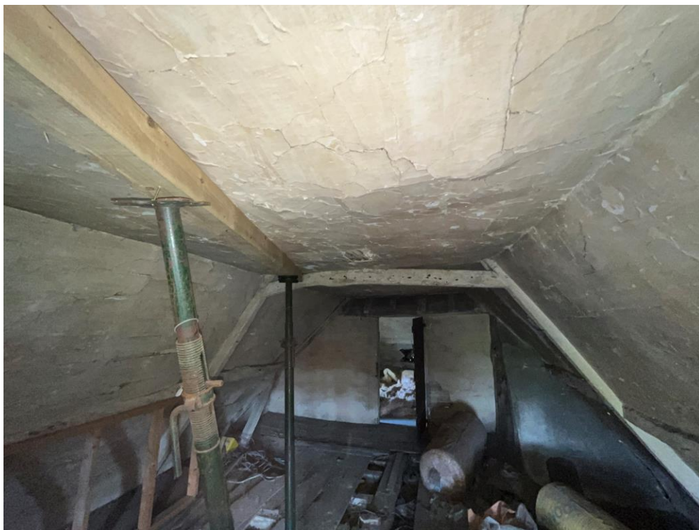
Propping to collars in roof space
