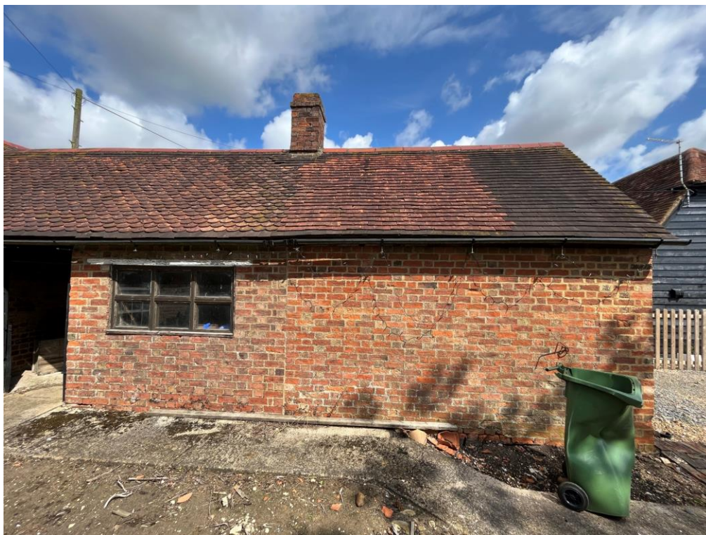
Storeroom roof externally, including mixture of tiles.
