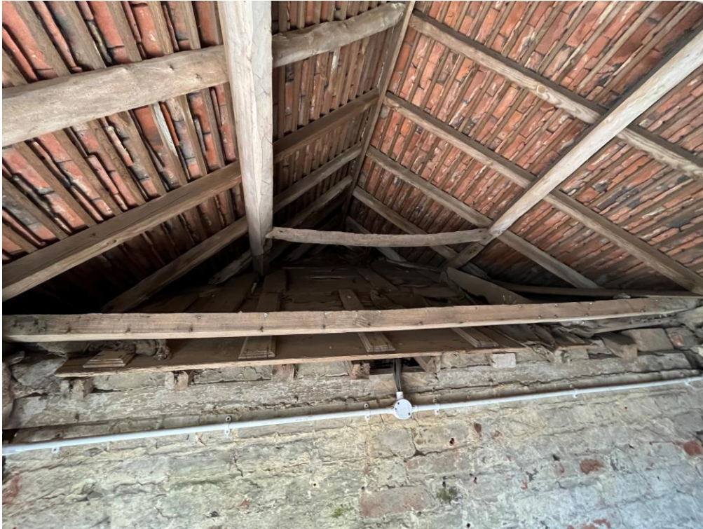
Over spanning purlins in forge.
