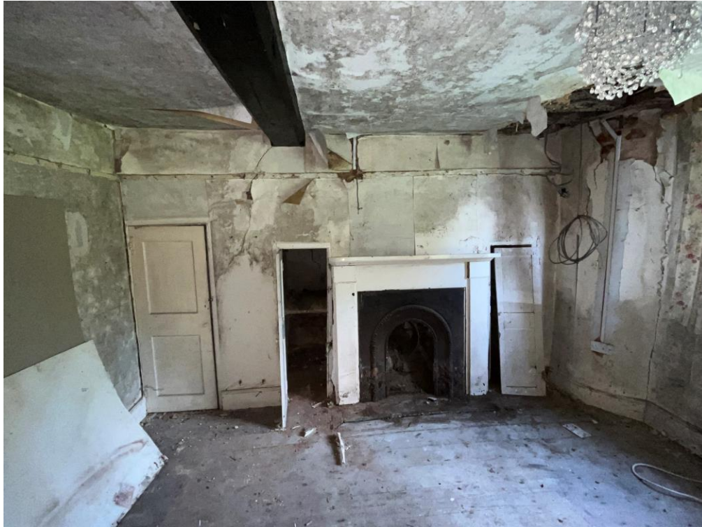
Southern Gable fireplace in drawing room.
