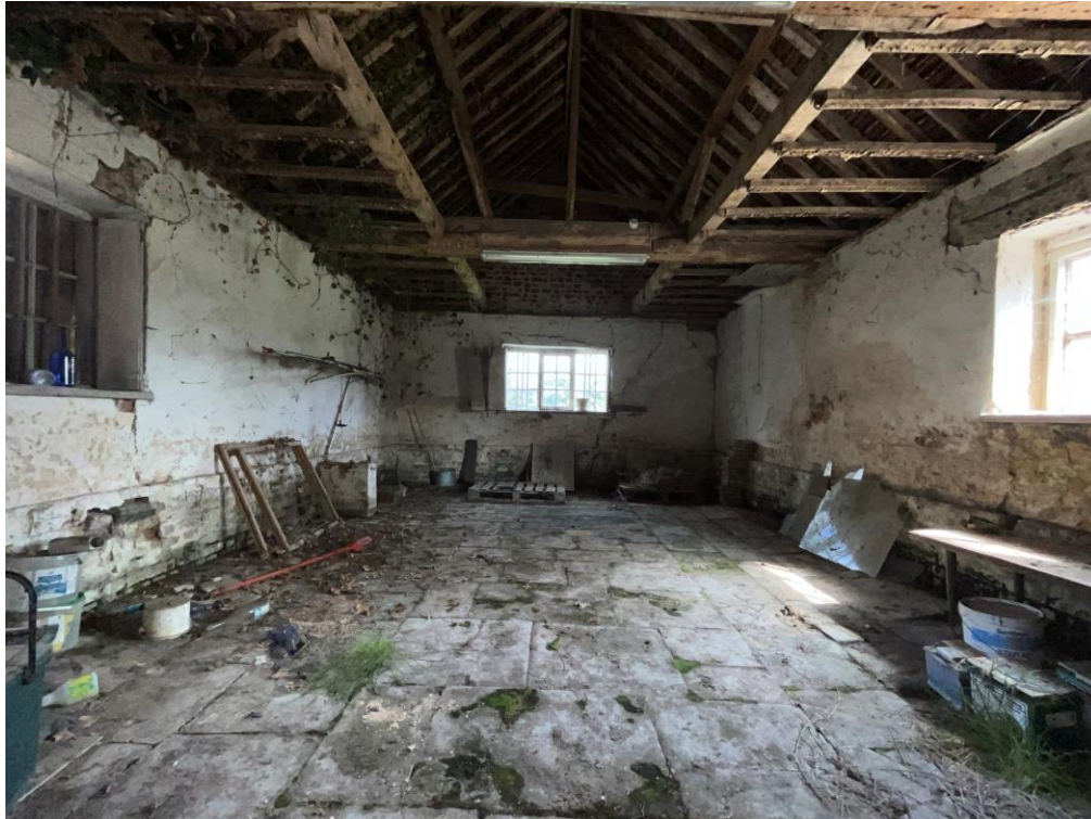
Inside the Dairy
