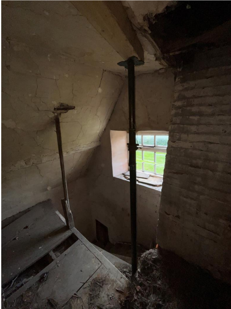
Propping roof space
