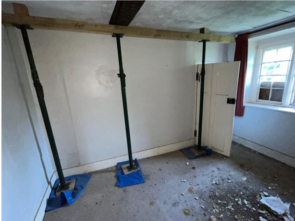
Propping to 2 nd floor.
