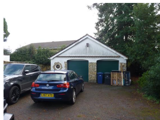
Views of front forecourt and garage of Ashley Pines
