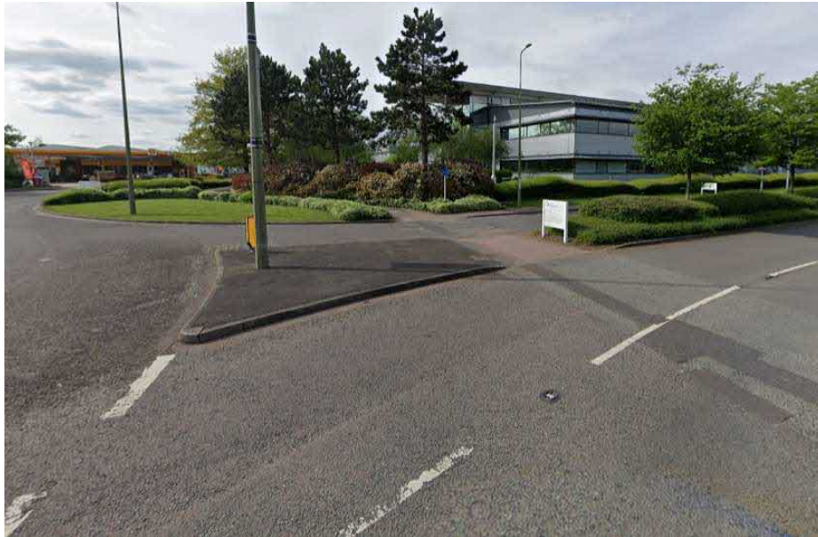
Photo 1: Pedestrian and cycle path on Garsington Rd. looking towards Cowley
