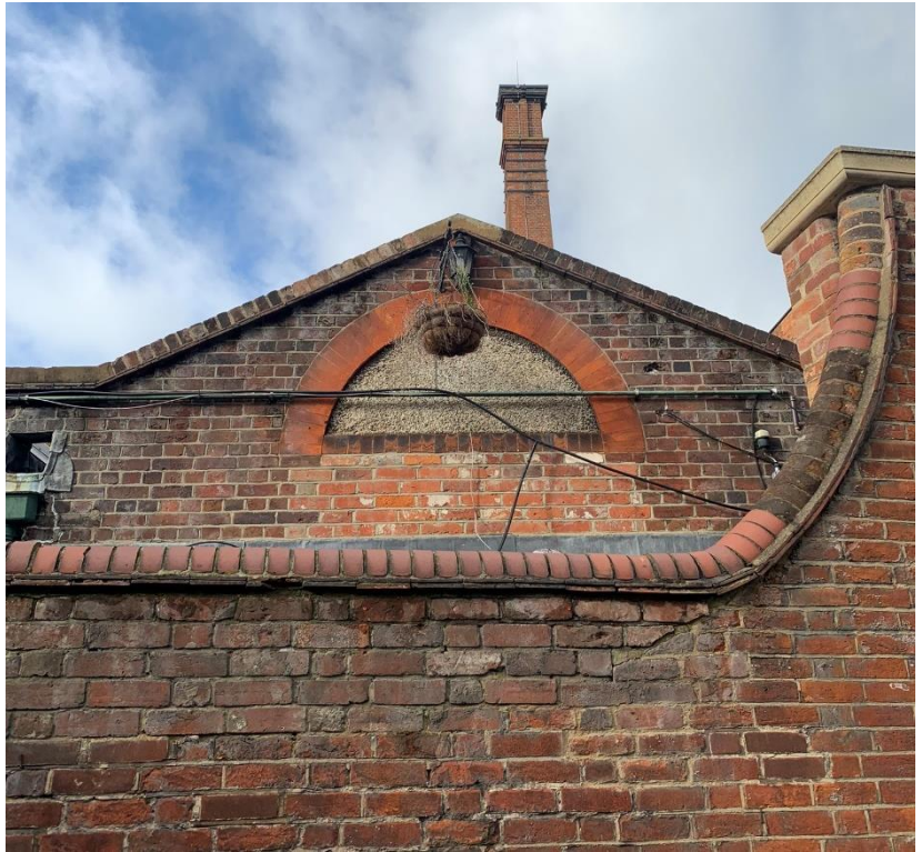
Figure 3 - External brickwork showing later alterations. (Survey Photo)
