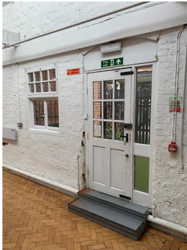
G.RM 10 – ROOM 5: Timber door replaced & new wall finish.
