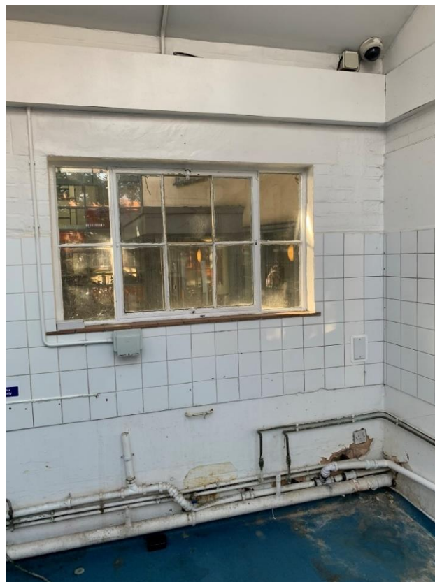
G.RM 01 - KITCHEN: Windows
