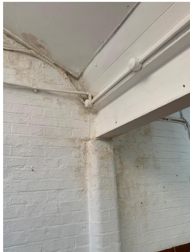
G.RM 08 – ROOM 4: Leaking roof repair & mould removed.
