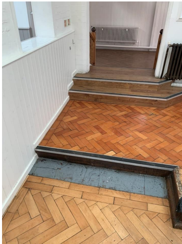
G.RM 08 – ROOM 4: Steps removed & new flooring.
