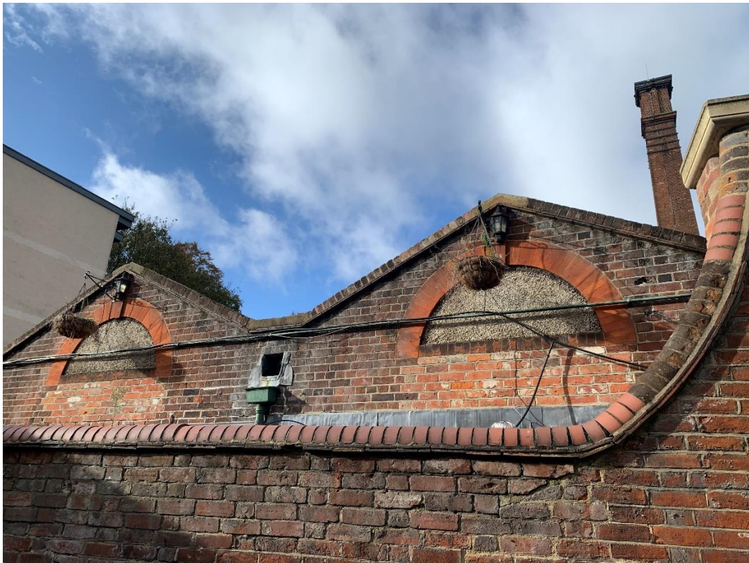
G.RM – STREET ELEVATION: Arch window opening made & bricks cleaned.
