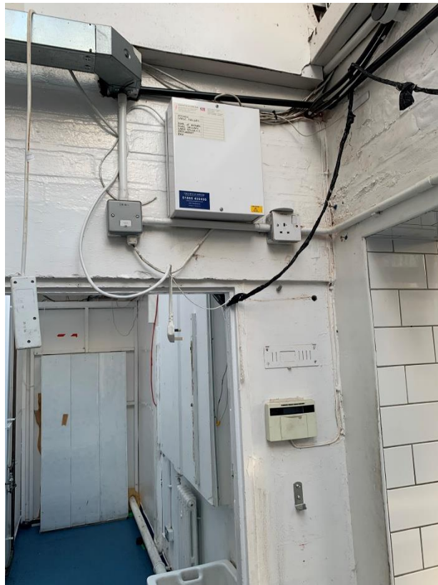
G.RM 01 – KITCHEN: Wall finish & cable tidy
