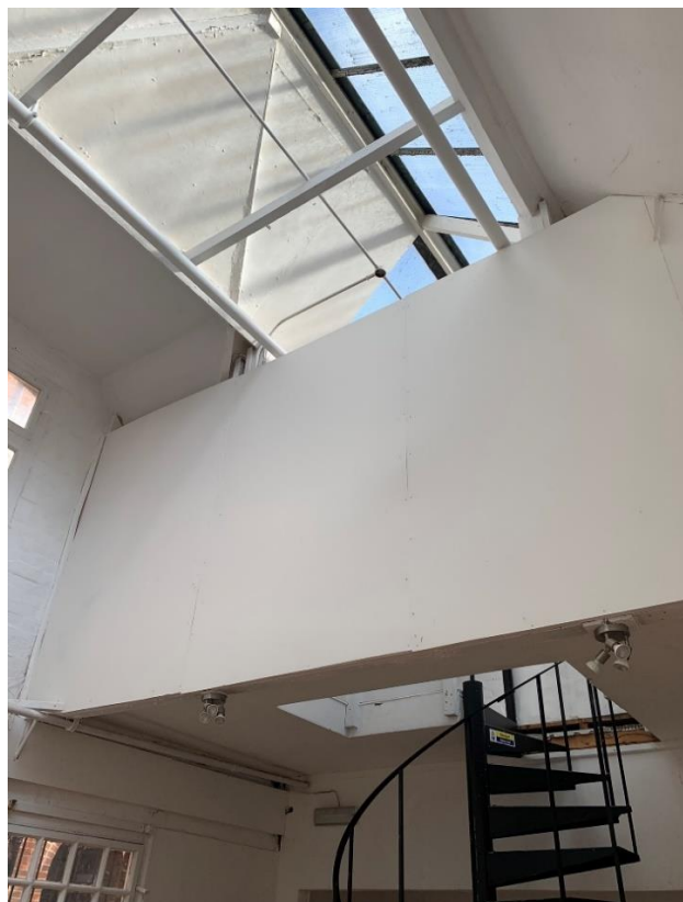
F.RM 01 – Mezzanine: mezzanine removed, & walls replastered.
