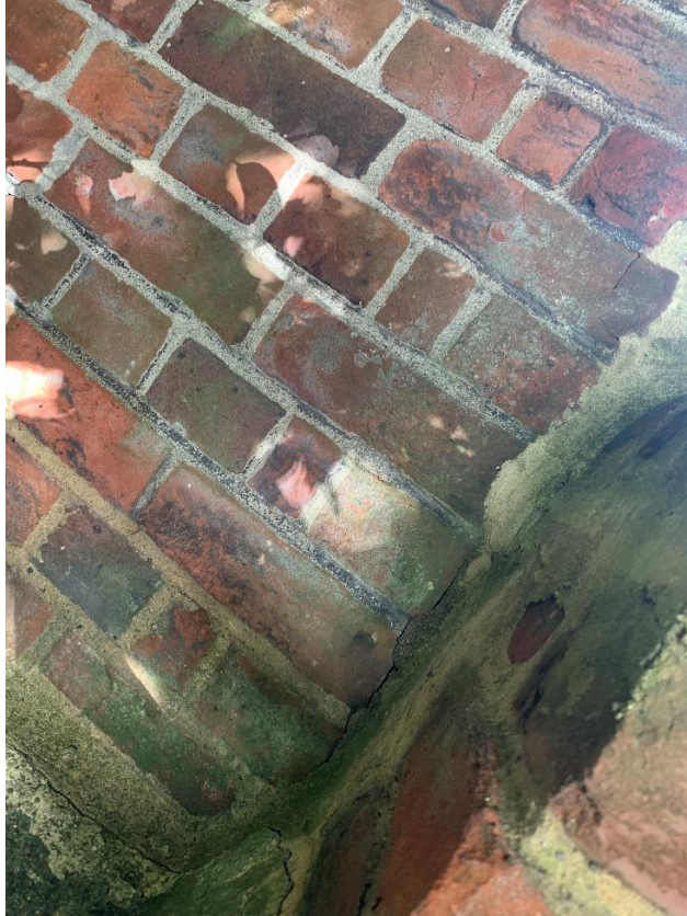
G.RM – External wall to be cleaned & repair where necessary.
