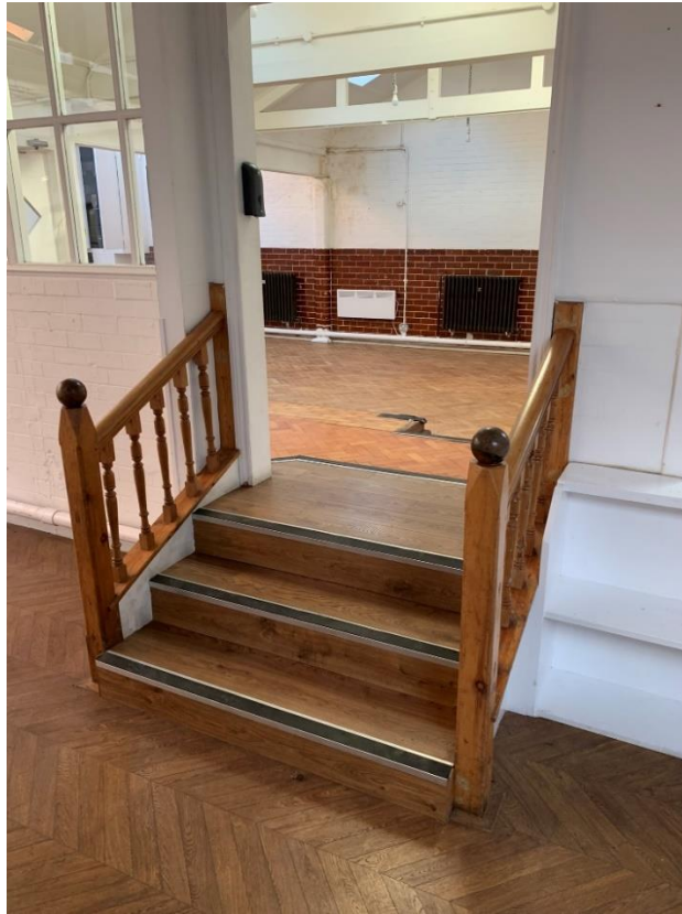
G.RM07 – ROOM 3: Steps removed & new flooring.
