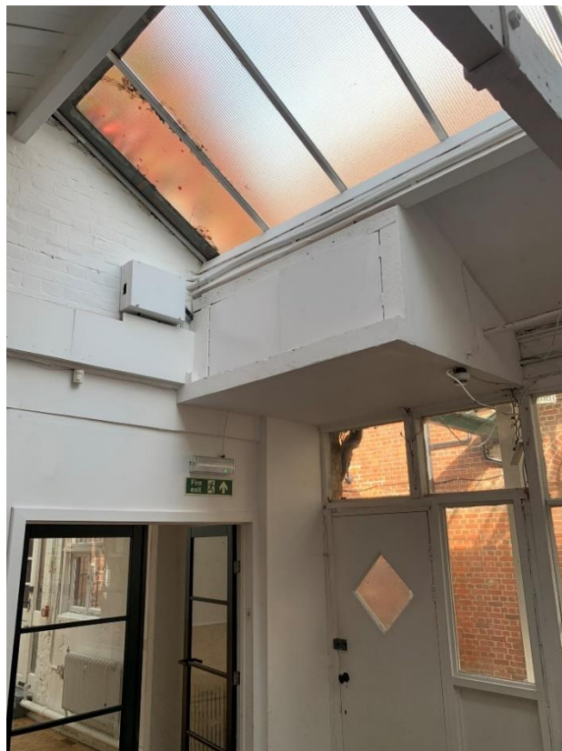
G.RM 07 – ROOM 3: Courtyard entrance to be repaired.
