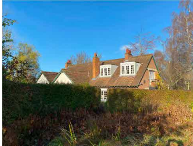
Figure 11: Oblique view of the south elevation of The Kilns
