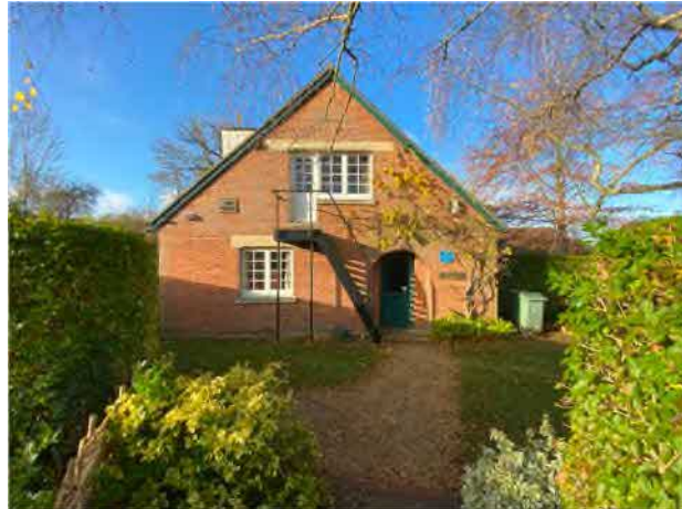
Figure 13: East elevation of The Kilns
