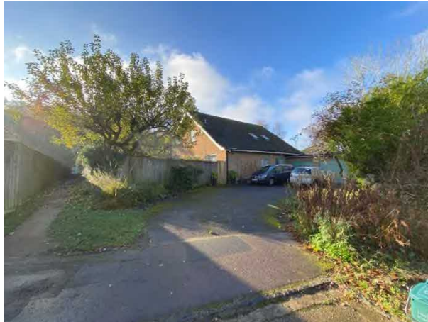
Figure 8: 8 Lewis Close viewed from the road
