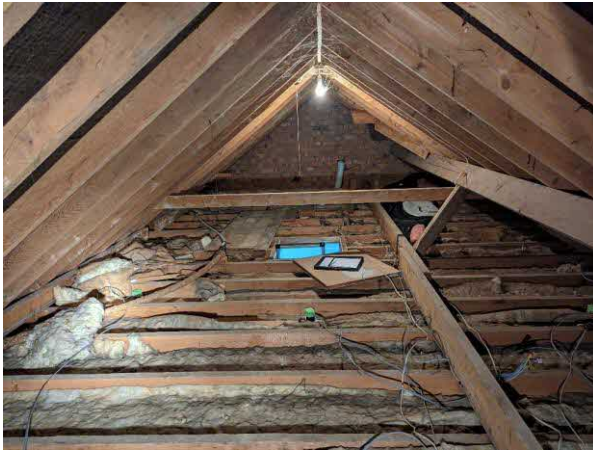
Photograph 3. Interior of the loft space.
