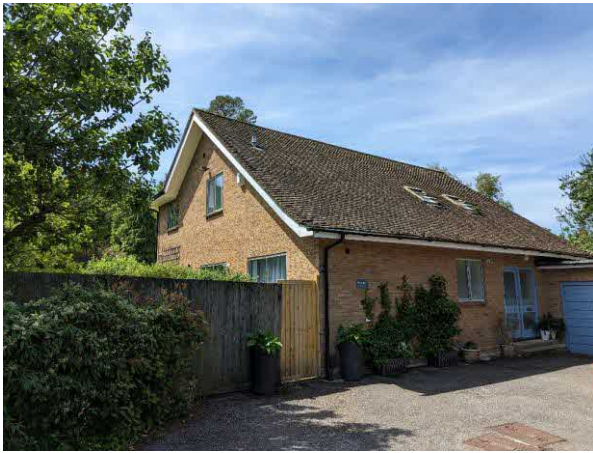
Photograph 1. The dwelling at 8 Lewis Close, viewed from the north-east.
