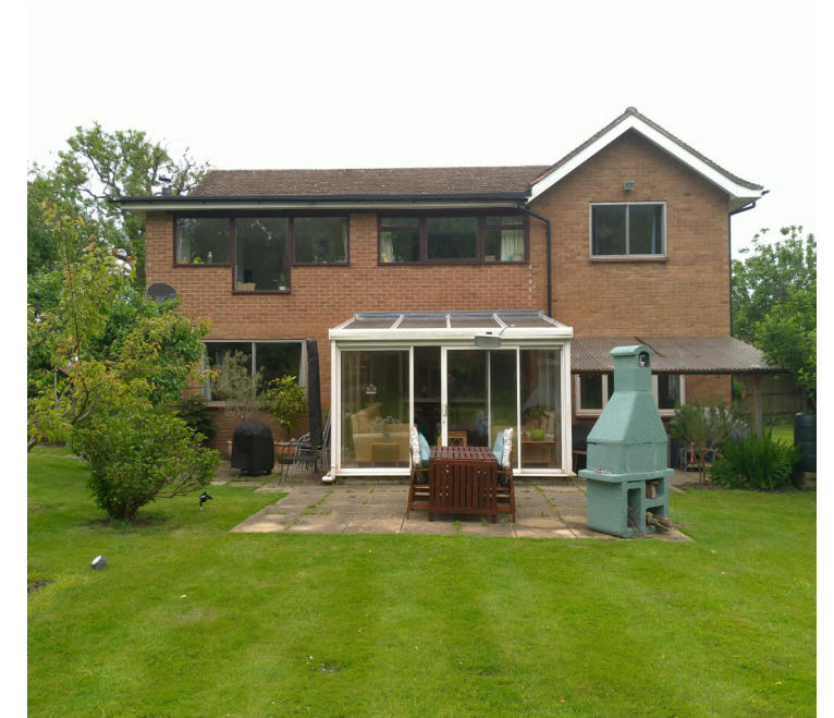
Rear Elevation of Existing House
