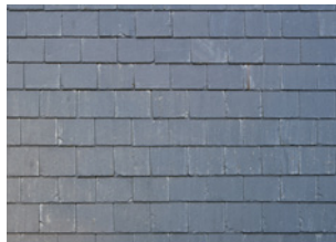
Grey Slate Roofing
