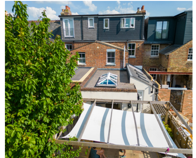
4. View of the rear elevation of the property
