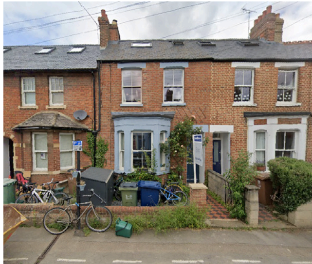
3. Image depicting the front elevation of the property
