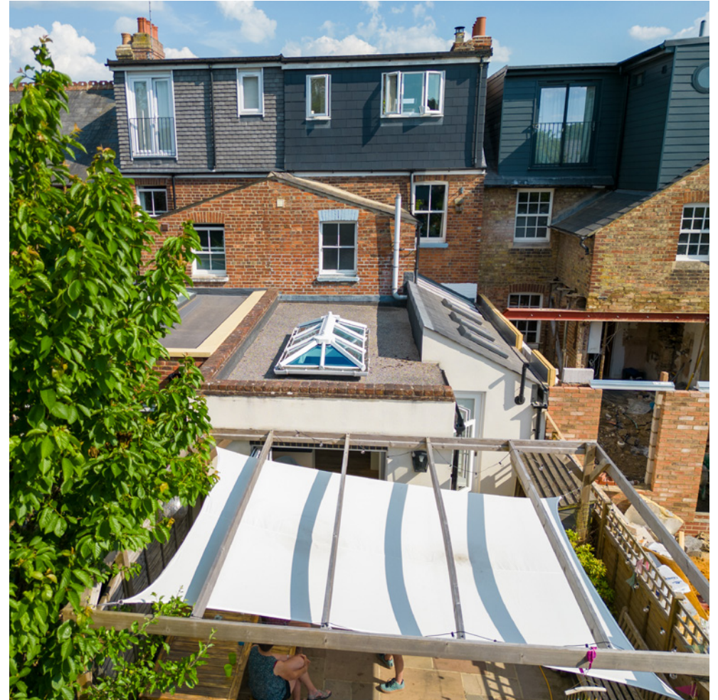
Rear Elevation (showing the existing rear extension)
