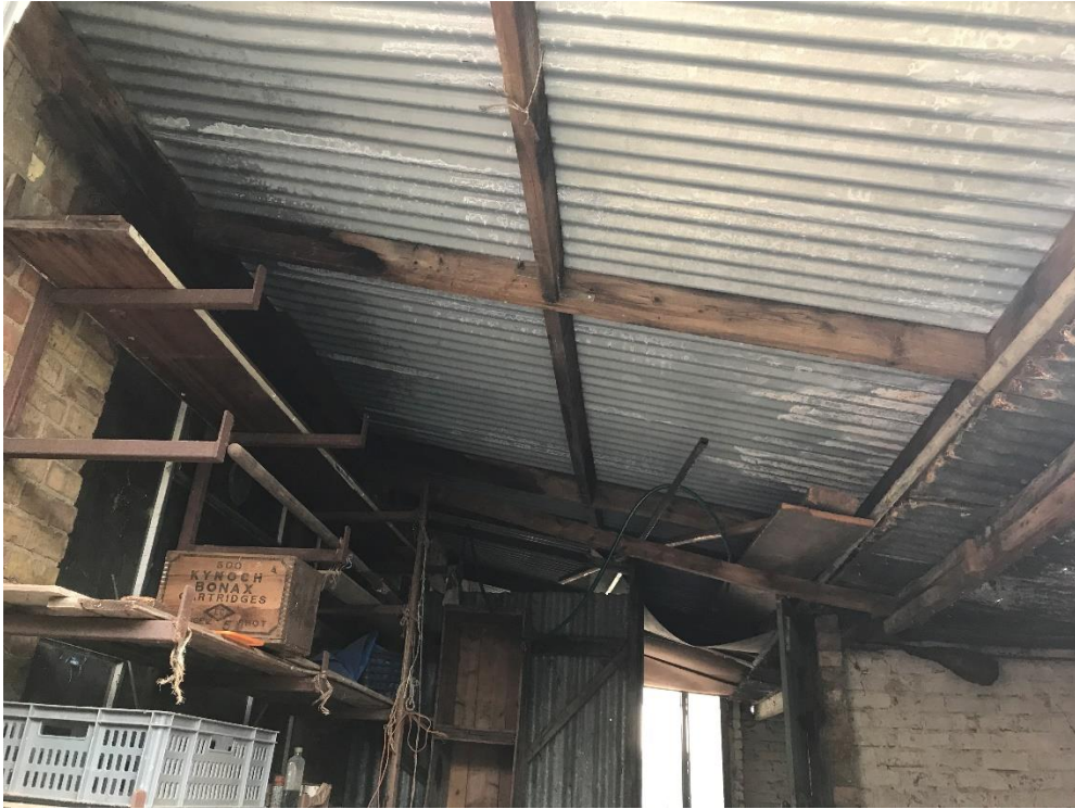
Photo 27 – Outbuilding, underside of east roof.
