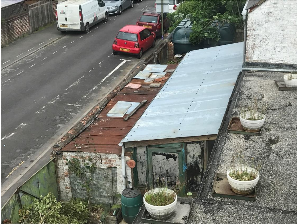
Photo 7 – Roof (s) of outbuilding.
