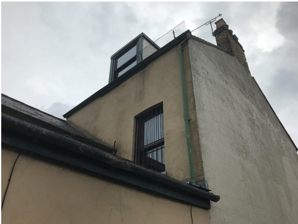
Photo 4 – Rear, north-west elevation.
