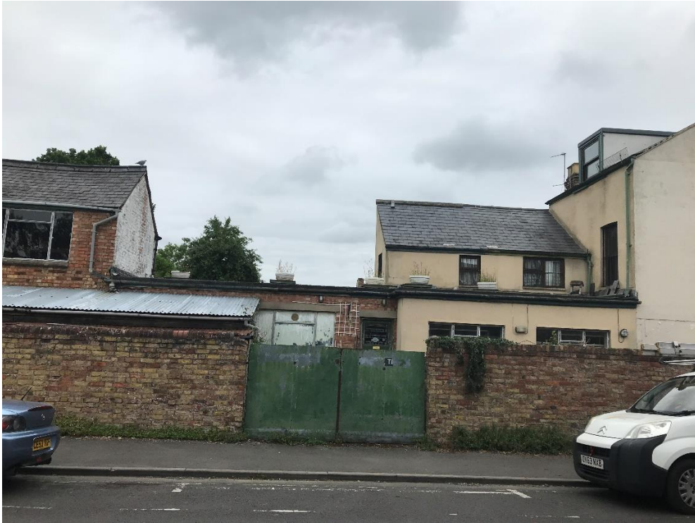
Photo 3 – Side, south-west elevation.
