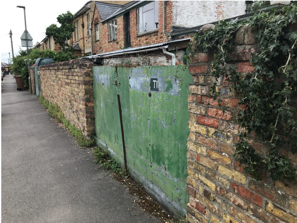
Photo 29 – South west boundary wall to Hurst Street.
