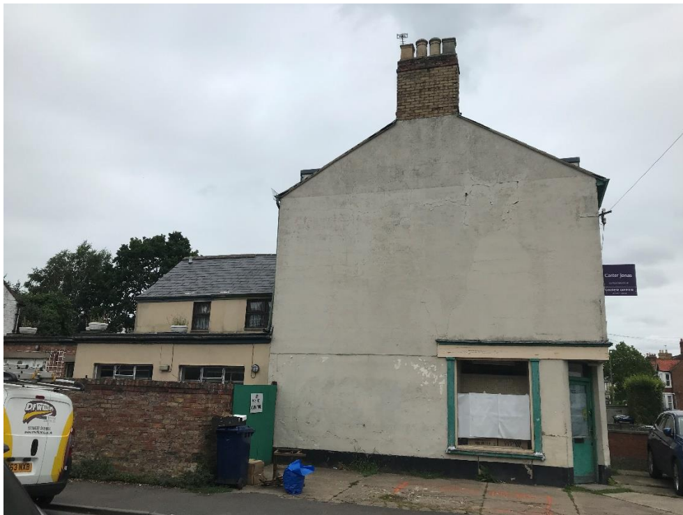
Photo 2 – Side, south-west elevation.
