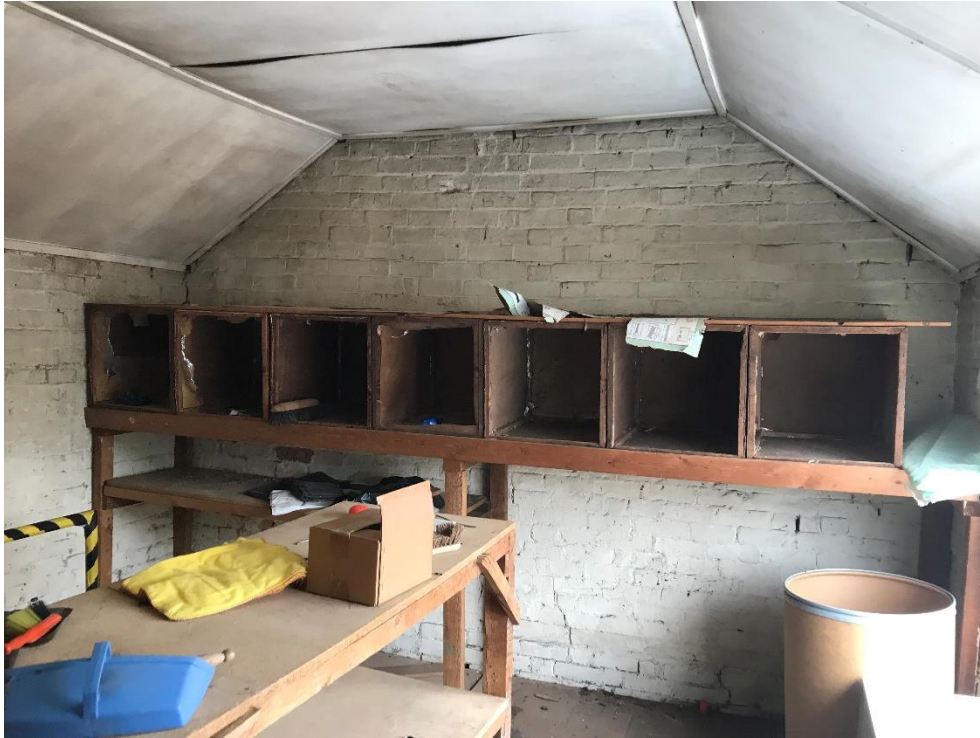
Photo 21 – Rear two storey building, first floor south.
