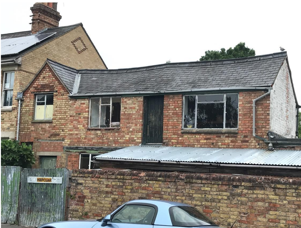
Photo 8 – South-west elevation, rear two storey building.
