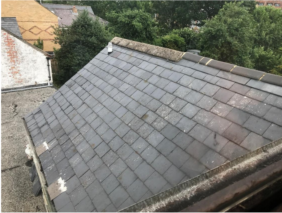
Photo 5 – Roof over original two storey section.
