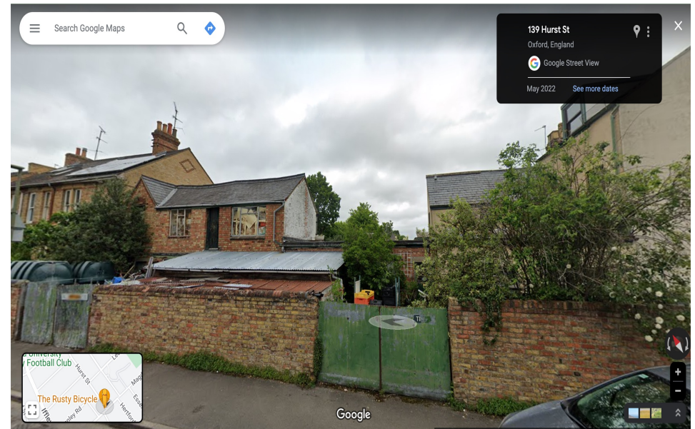
Back of Shop (right) with with flat above, with outbuildings used as stores for the shop behind (Left). 2x Parafin tanks visible on far left. View from Hurst Street.
