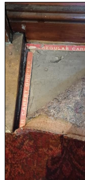
Figure 5: Concrete Floor Under Carpet
