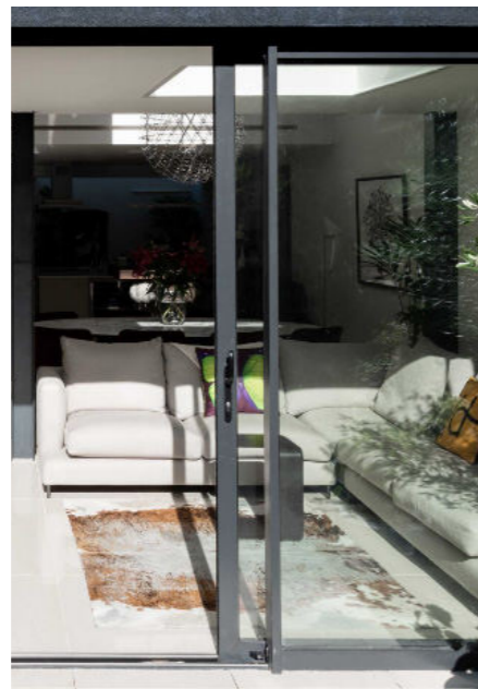
Triple glazed thin-frame aluminium sliding glass doors connect rear extension to back garden
