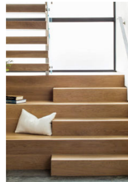
Dual height stair connecting extension to main house structure
