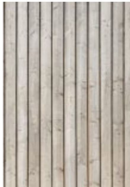
Light timber cladding over roof and walls of extension second floor
