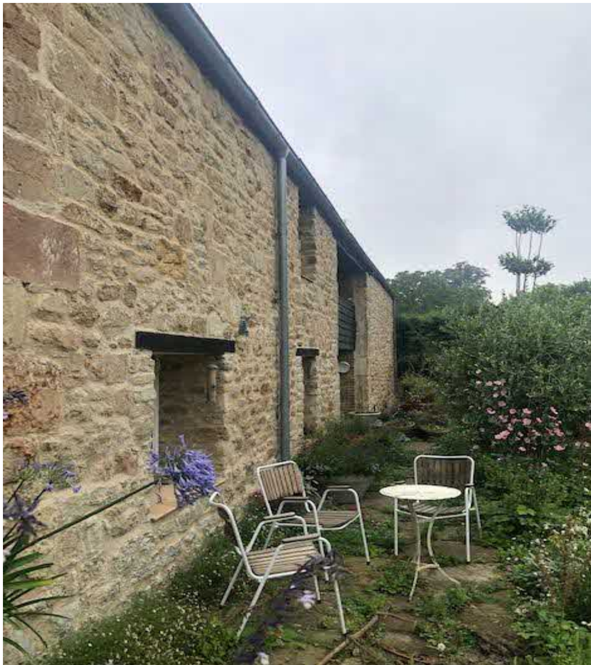
Figure 5 The Barn frontage onto the garden
