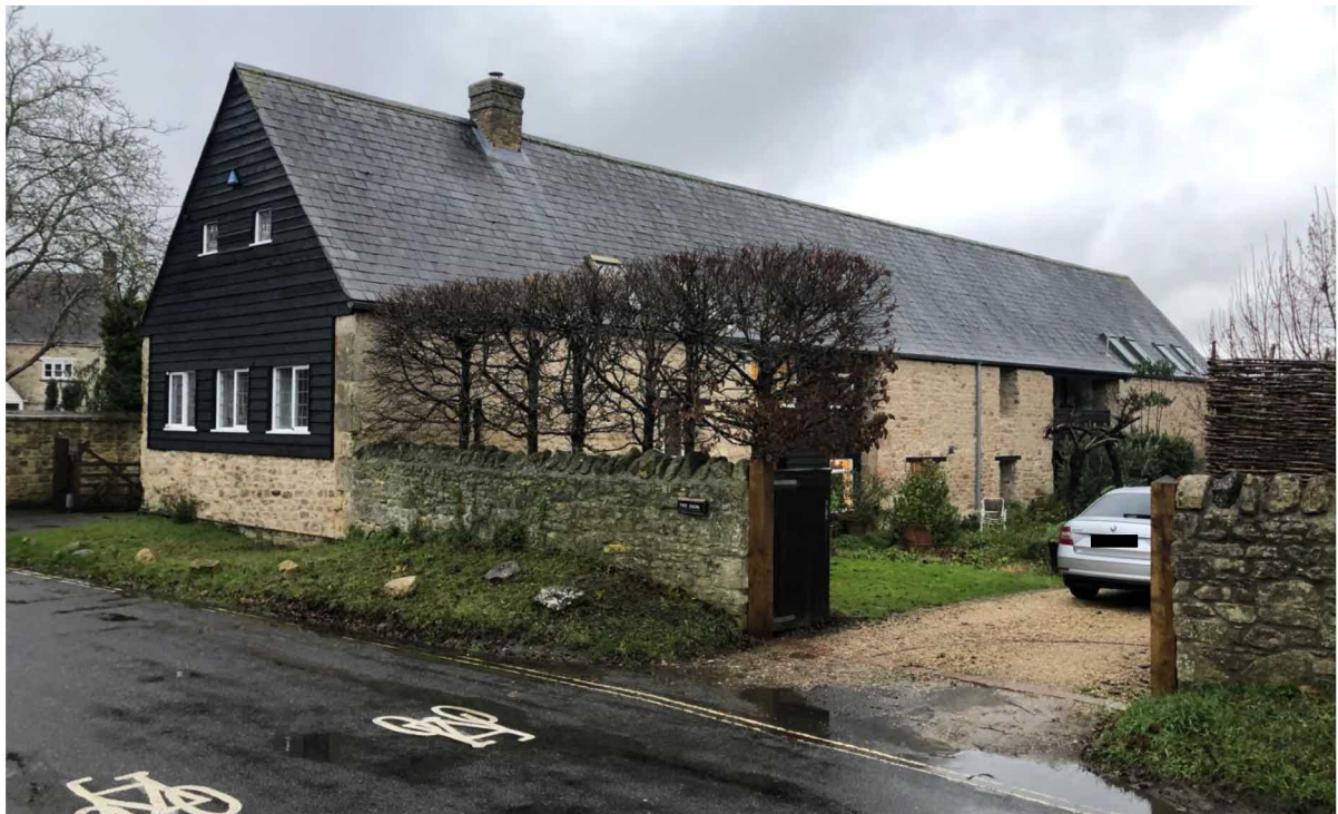
Figure 4 Entrance from Barton Lane
